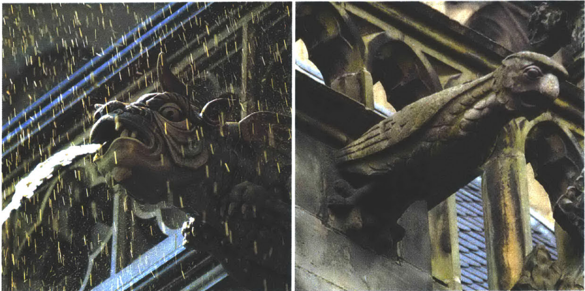
Figure 10.2: The photograph on the left from Crist [2001] shows a gargoyle downspout directing rainwater away from the building. In the right image, from Benton [1997], staining and lichen growth from years of exposure are apparent on the gargoyle and the other architectural elements.
