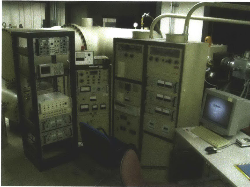
Figure 3-8: Photo of the new arrangement of the tandem accelerator controls
