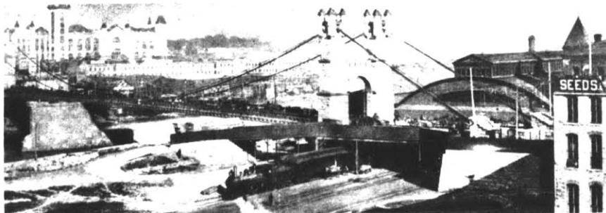
STEEL SUSPENSION BRIDGE BUILT IN 1879 TO REPLACE WOODEN SPAN ABOVE
