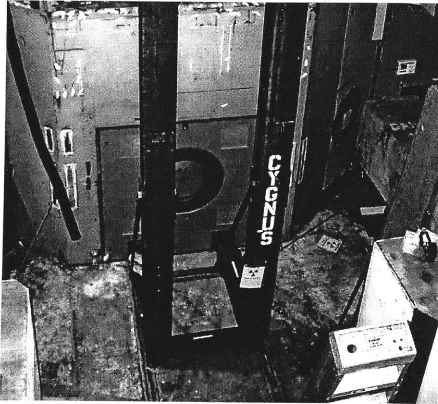
2-04 Photograph of the area outside of the Water shutter and Collimator where the Mechanical Shutter will be installed
