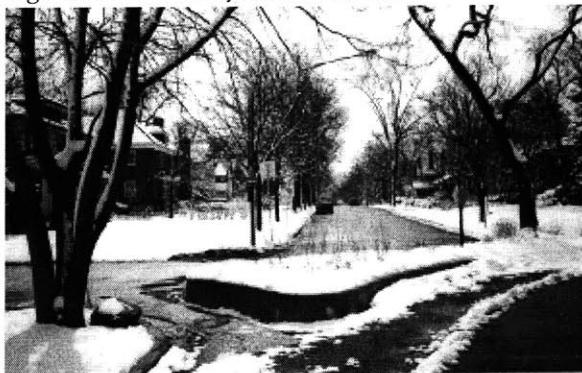
Fig 6.8. North Beverly internal diverter.
