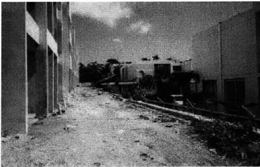
Fig 2.16. Edge condition between new multi-family amoeba and adjacent neighborhood near Torrimar station.
