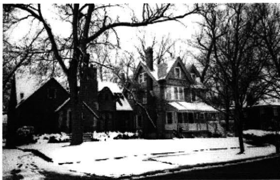
Fig 6.3. Typical North Beverly streetscape
