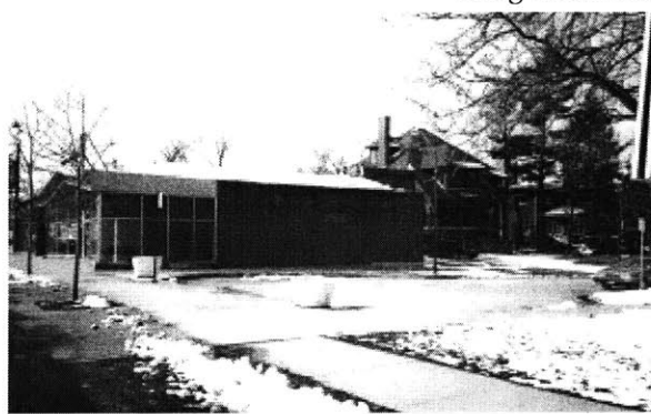
Fig 6.9. Continuous sidewalk cul-de-sac along 95th Street.
