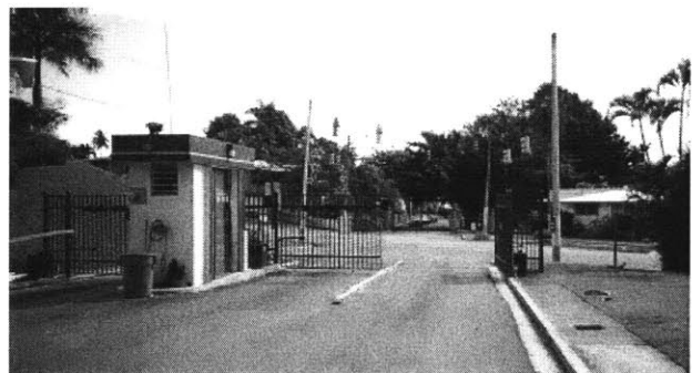
Fig 2.4. Note gate blocking sidewalk on right, but adjacent unblocked front lawn.
