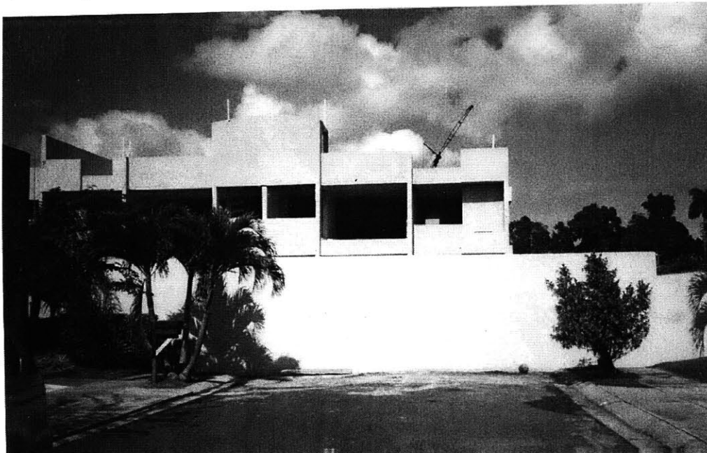
Fig 2.18. Street in existing neighborhood sealed off with wall and rear of new multi-family amoeba.
