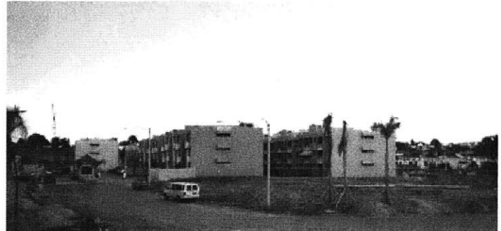
Fig 2.17. View of multi-family amoeba under construction near Torrimar station.
