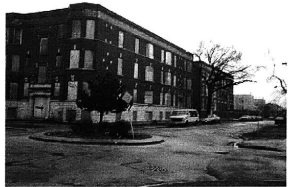
Fig 6.18. North Lawndale landscaped traffic circle.
