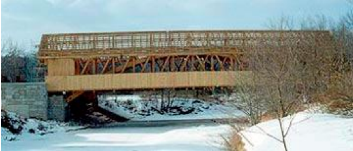
Figure 4.1: Smith Millennium Bridge ( gratonconst.com )
