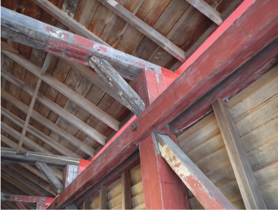
Figure A 27: Barrackville Bridge Bracing Support Detail
