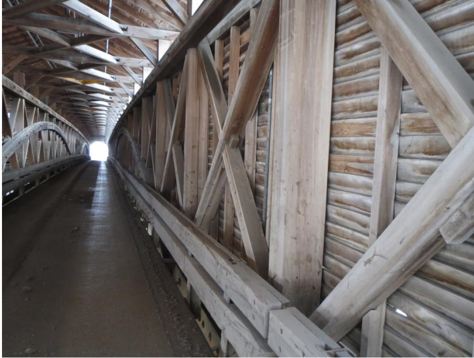
Figure A 29: Interior Long Truss framing, Philippi Bridge
