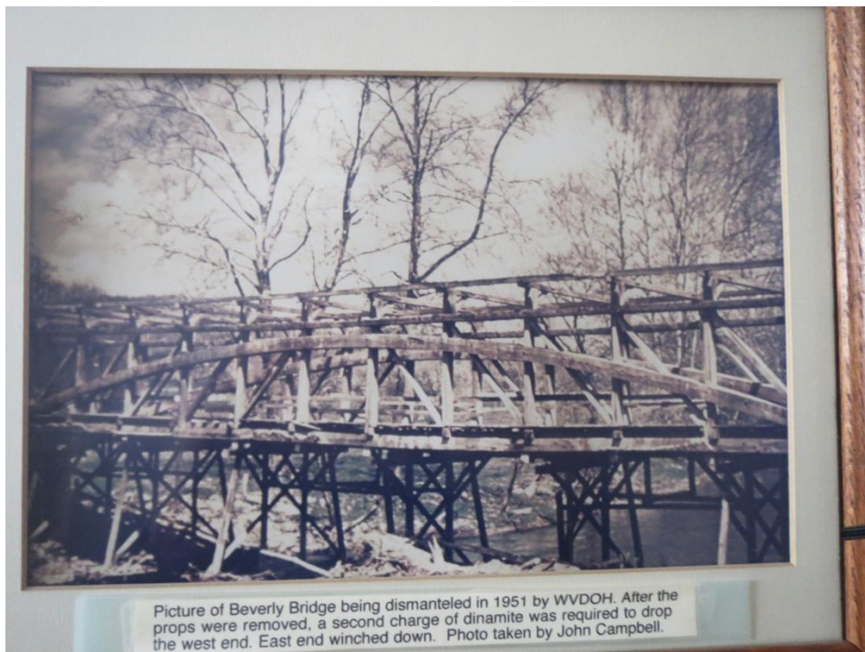
Figure A 7: Beverly Bridge Immediately Prior to Demolition, photo courtesy of Randy Allan
