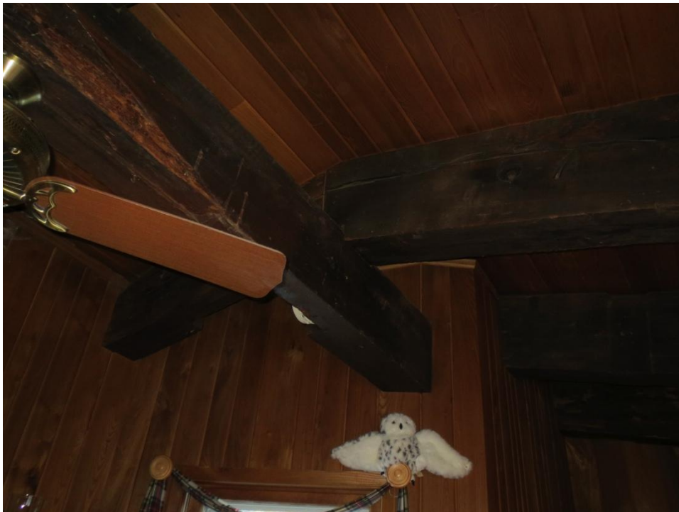
Figure A 9: Salvaged Beverly Bridge Timbers
