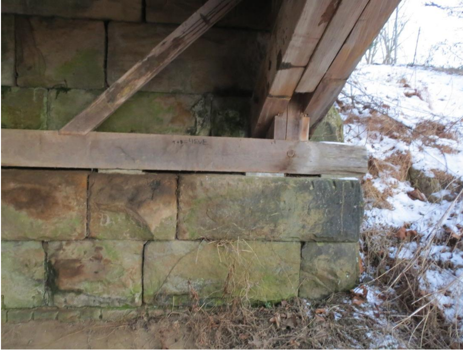
Figure A 21: Arch Landing of Barrackville Bridge
