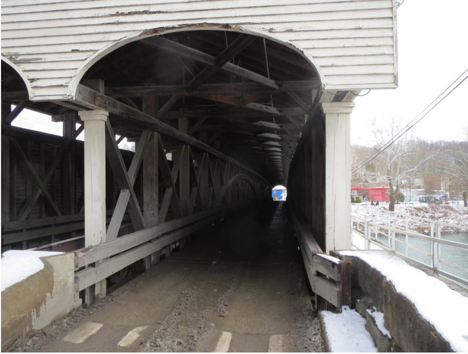
Figure A 31: Philippi Bridge Portal, showing the concrete deck and guardrails
