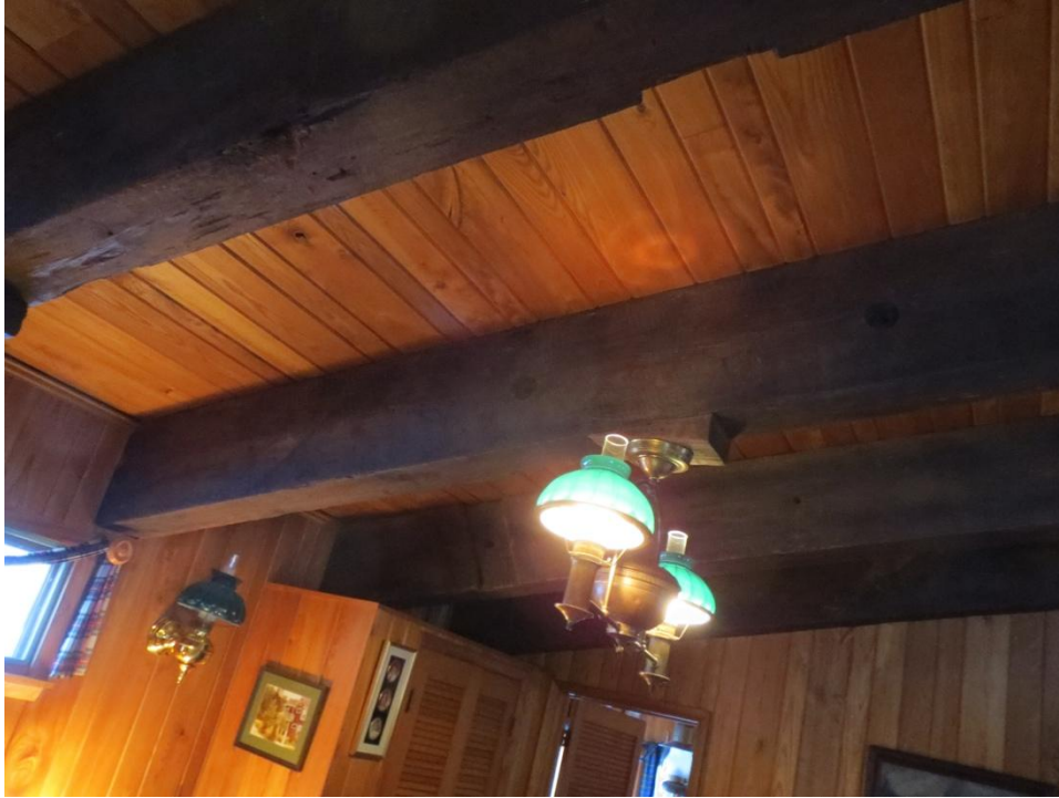
Figure A 10: Salvaged Beverly Bridge Timbers
