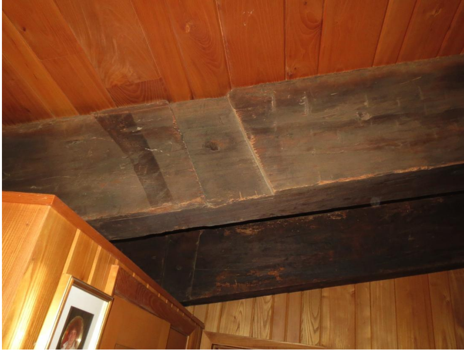
Figure A 8: Salvaged Beverly Bridge Timbers
