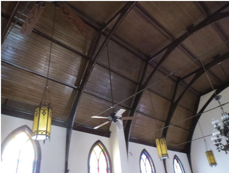
Figure A 19: Roof Structure of Tygarts Valley Presbyterian Church
