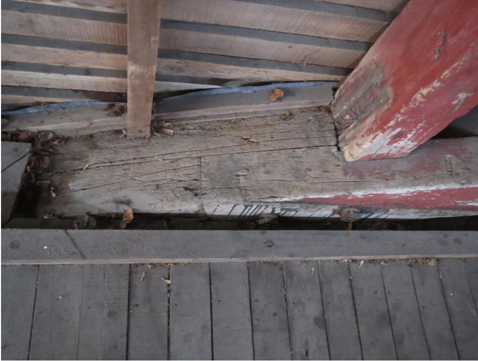
Figure A 25: Half-Lap Arch Splice, Barrackville Bridge
