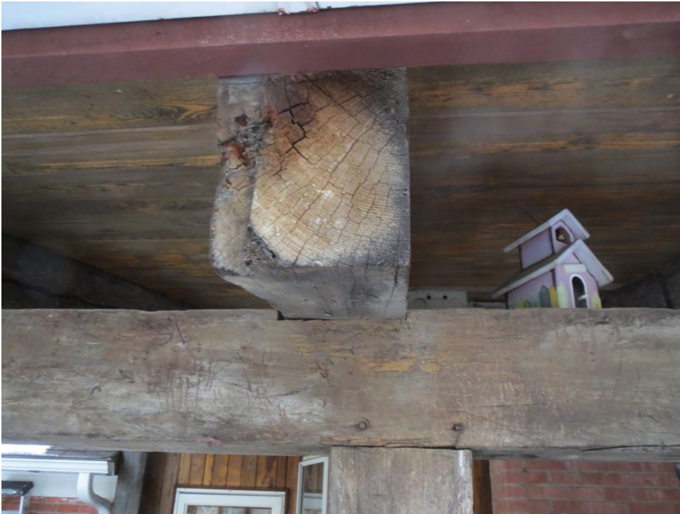
Figure A 15: Salvaged Beverly Bridge Timbers, showing growth rings of the member
