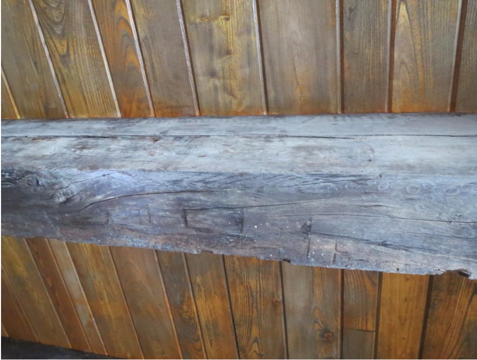
Figure A 16: Salvaged Beverly Bridge Timbers, showing axe marks
