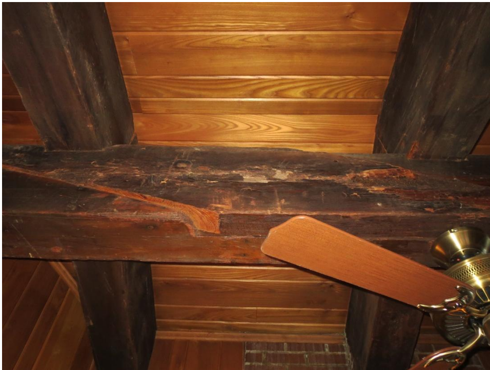
Figure A 11: Salvaged Beverly Bridge Timbers
