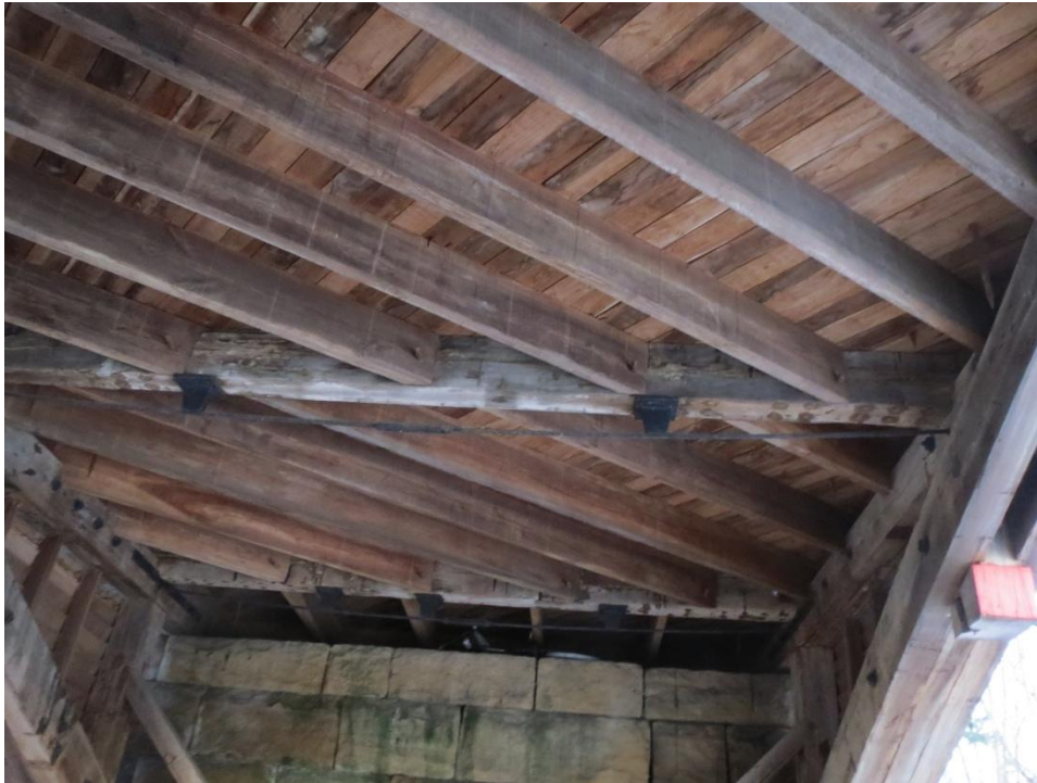
Figure 2.8: Barrackville Floor Framing (photograph by author, 2014)
