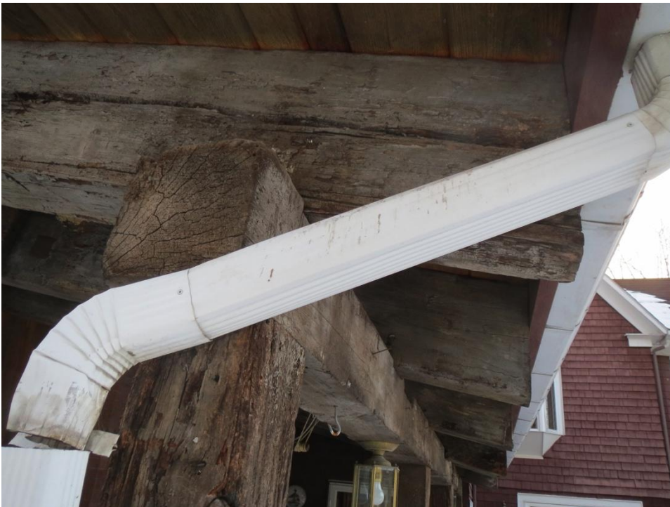
Figure A 17: Salvaged Beverly Bridge Timbers
