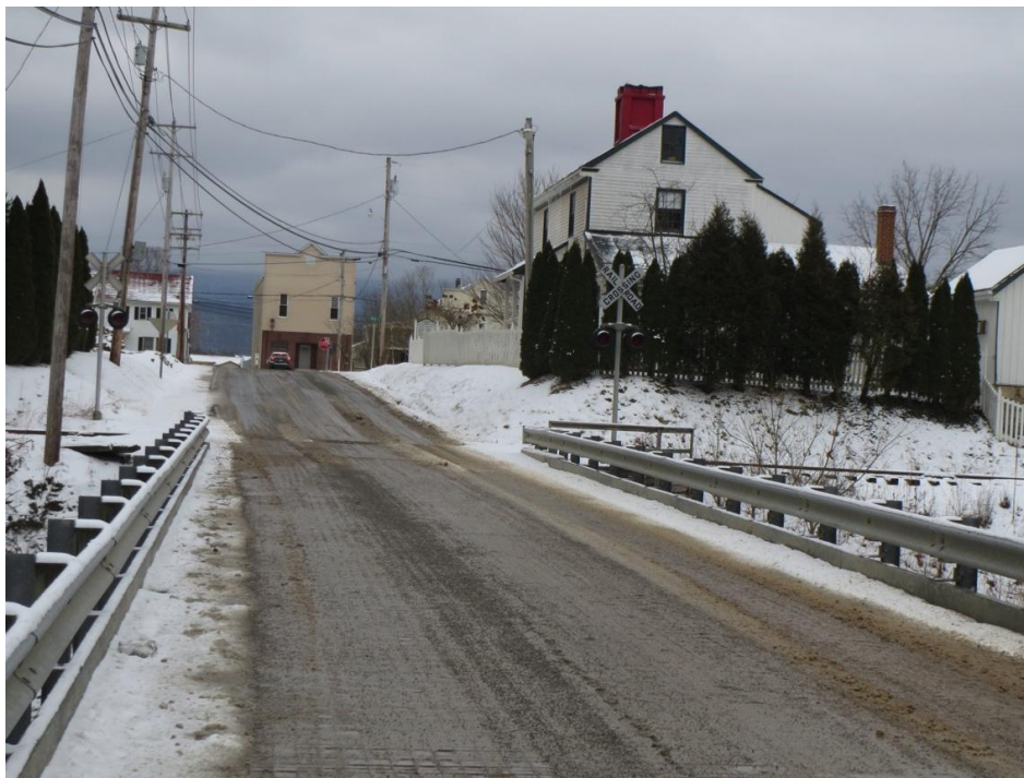
Figure 2.2 Current Beverly Bridge Roadway, with Chenoweth's House on right (photograph by author, 2014)
