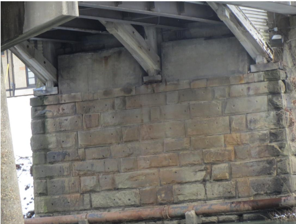
Figure A 28: Arch Landings and Abutments, Philippi Bridge
