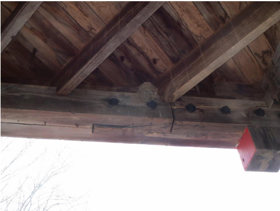
Figure A 22: Bottom Chord Splice of Barrackville Bridge
