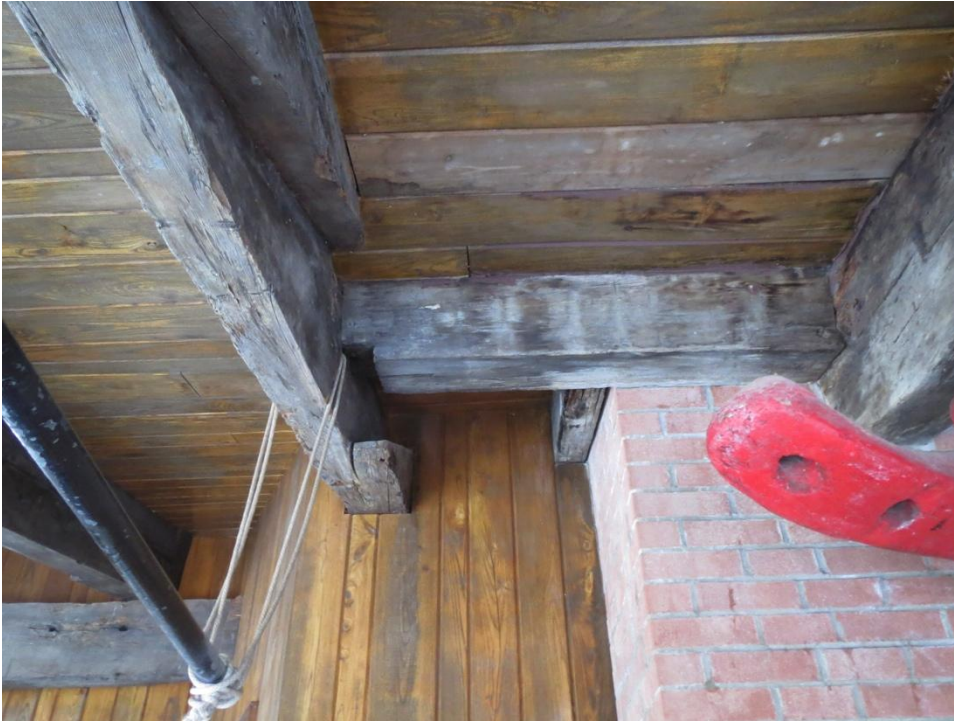
Figure A 14: Salvaged Beverly Bridge Timbers
