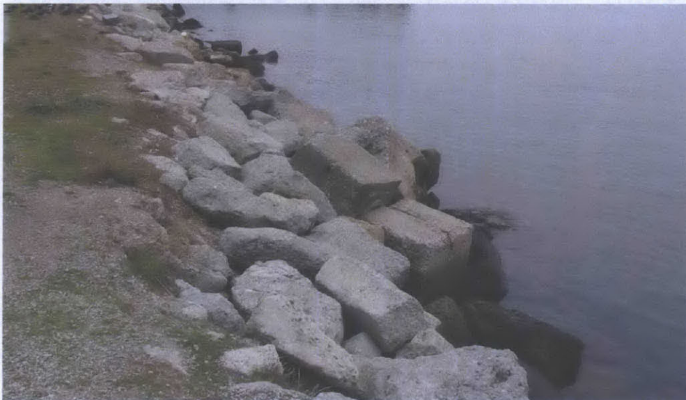
FIGURE 14: STONE REVETMENTS (IXIGO.COM, N.D.)
