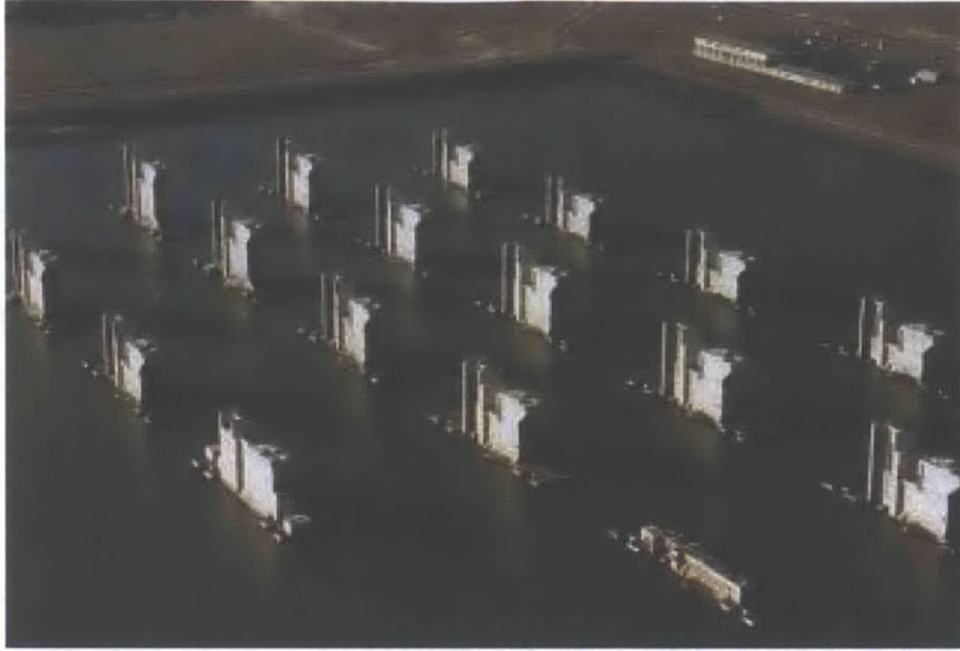
FIGURE 12: PIER SYSTEM UNDER CONSTRUCTION (DELTAWERKEN ONLINE, 2004)
