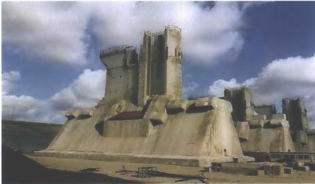
FIGURE 13: CONSTRUCTION OF PIER (DELTAWERKEN ONLINE, 2004)
