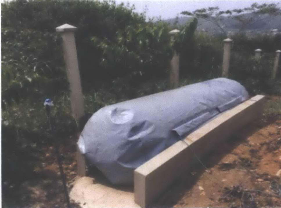
Figure 1-14 Ashesi University's methane collection system, attached to their anaerobic digester
