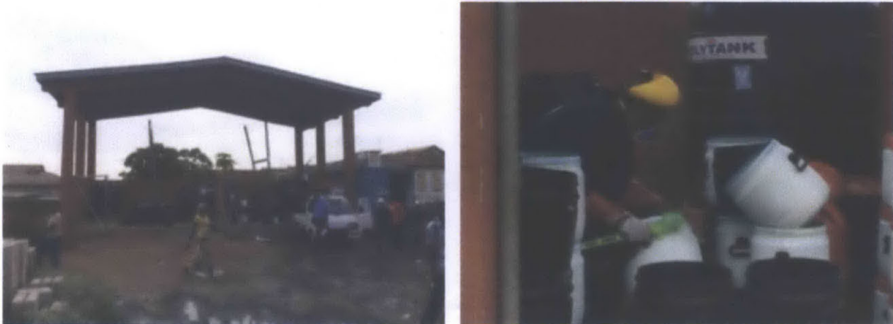
Figure 3-5 The central processing location. Here, buckets are emptied into polytanks for holding until a vacuum truck transports the sludge to Dompouse. Clean Team members disinfect the buckets before recirculation.
