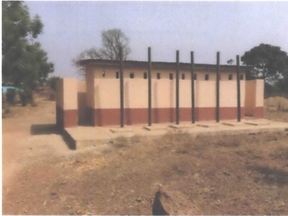
Figure 1-13 Taha pour-flush school block
