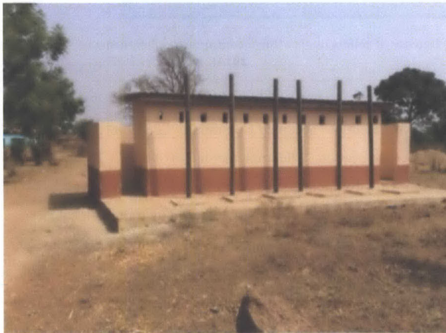
Figure 6-5 Exterior of the Taha Pour Flush Sanitation Facility
