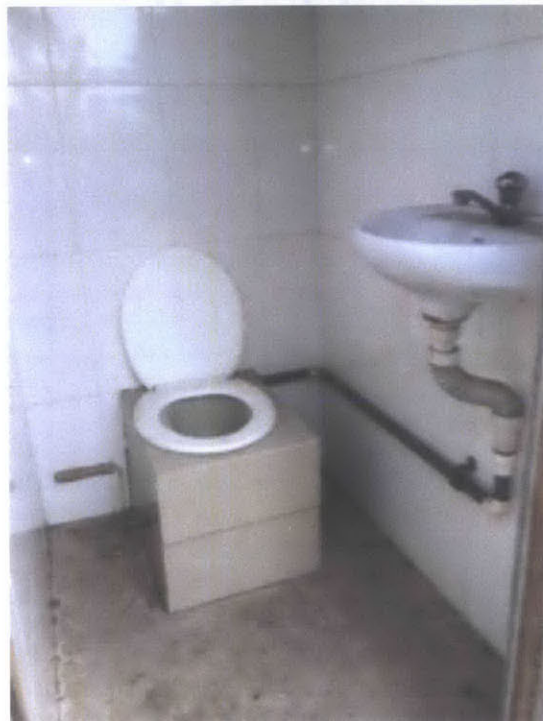
Figure 5-9 The interior of a Biofil Toilet
