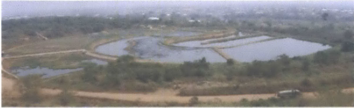
Figure 3-10 The waste stabilization ponds at Dompase in Kumasi (Tanner 2013)
