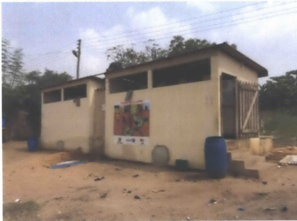
Figure 5-11 The public MFBF facility in Pokuase, constructed through a partnership of GSAP and Kweku Anno
