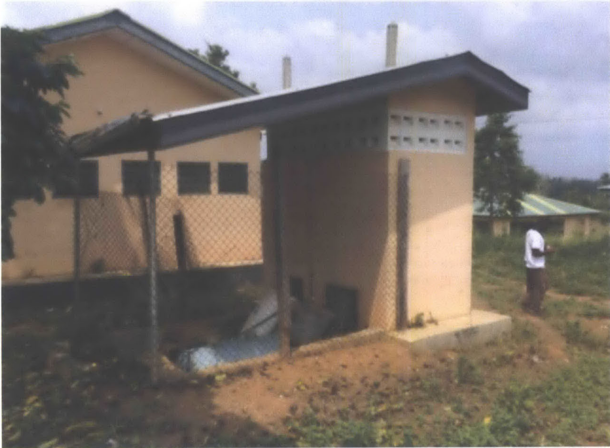
Figure 4-1 The MFCL at Nyastech Secondary School. Behind the latrine is a below grade area that houses the nitrification, anode, and cathode tanks, and next to the latrine is a newly built facility with flushing toilets.
