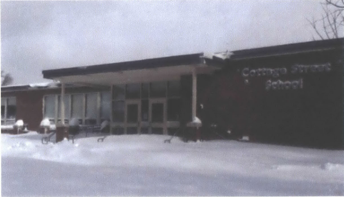
Figure 3-1: Cottage Elementary School in Sharon, MA
