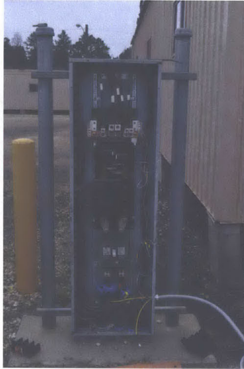
Figure 4-7: DepNILM installation at Ft. Polk FOB
