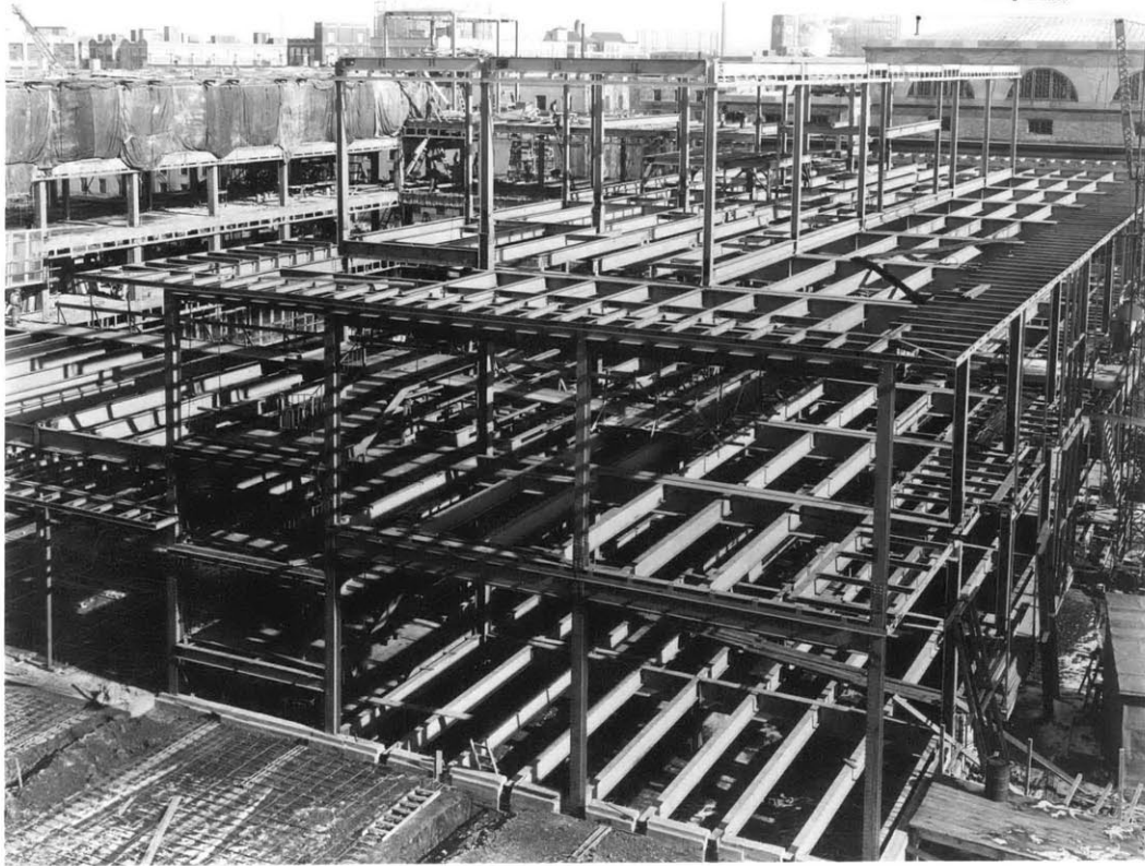
CHARLES HAYDEN MEMORIAL LIBRARY Progress Picture #19 Feb. 3, 1949 Facing Northeast.
