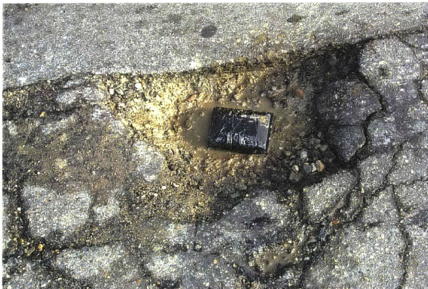
Photo 9: The Installed Node
