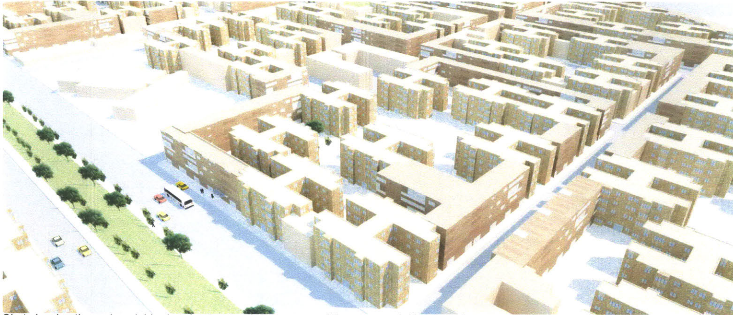
Shot showing the main neighborhood entrance, the mosque and the commercial boulevard
