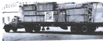
239 A special truck transports all the prefabricated panels for a small one-family house, including built-in units and kitchen and bathroom fixtures, to building sites within a radius of up to 300 miles. The horizontal boom mounted to the rear of the truck is used to place the individual groups of building elements at strategic points around the site.
