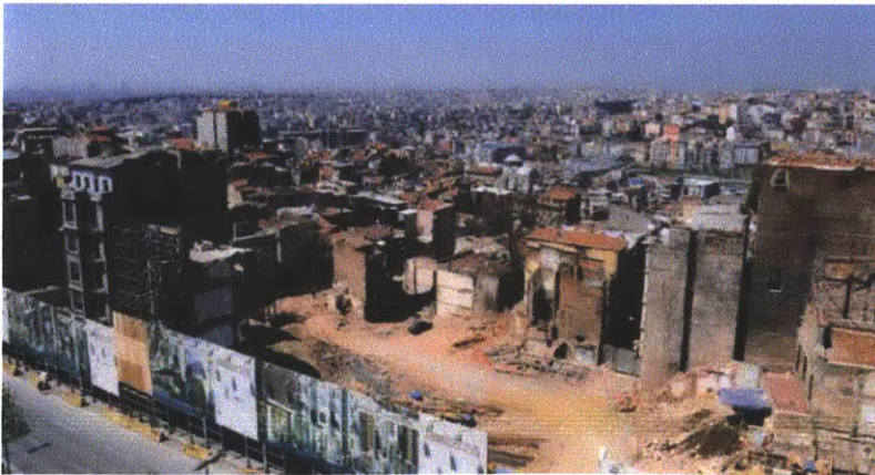
Figure 19. Tarlabasi urban renewal proposal under construction
