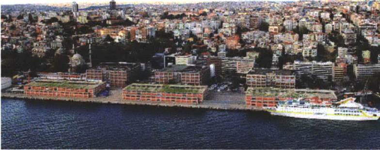
Figure 13. Historical warehouses under urban renewal transformation
