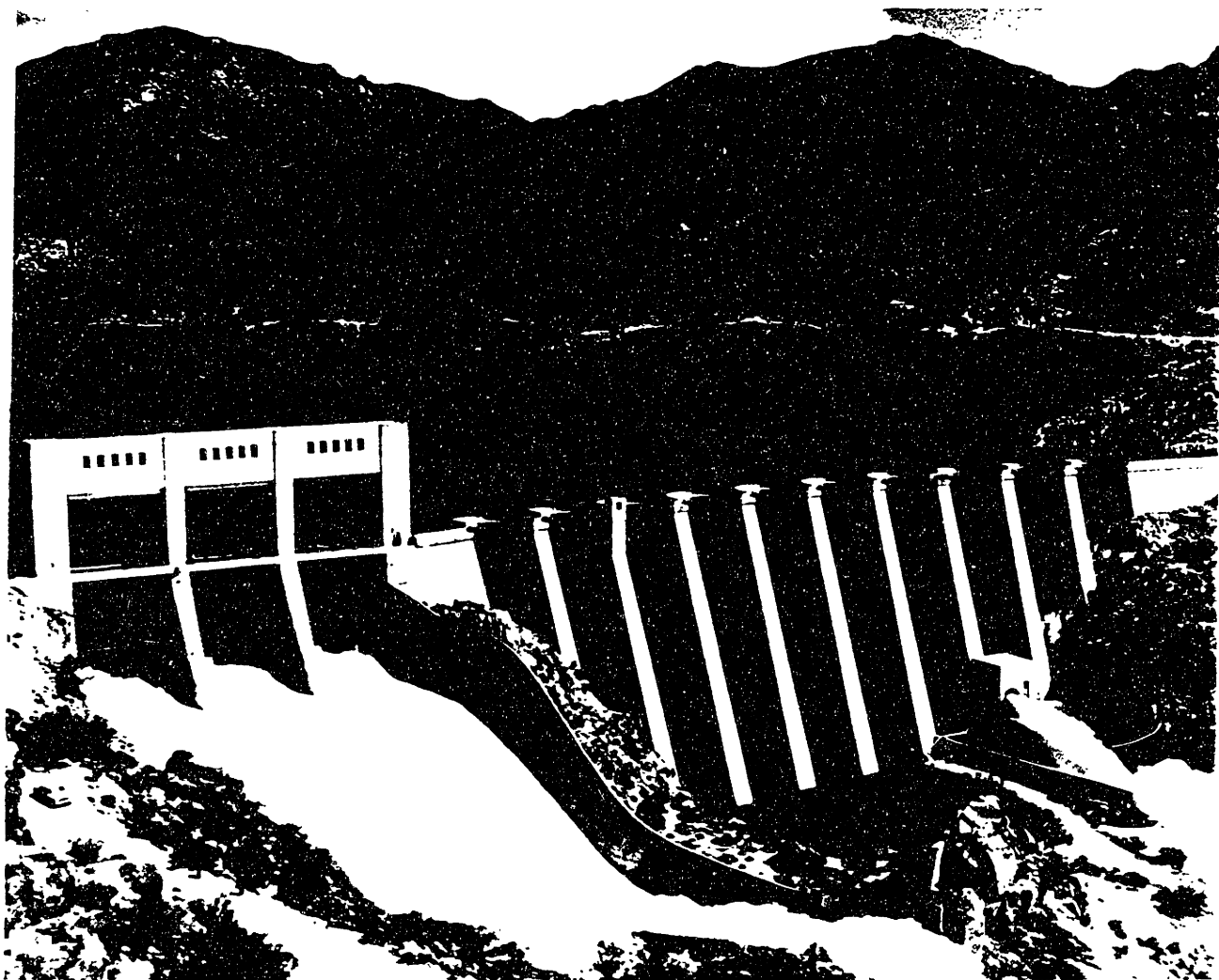
8.9 Bartlett Dam, north of Phoenix, Arizona, completed in 1939. This double-walled, hollow buttress structure was the only major multiple arch dam ever built by the Bureau of Reclamation. (Salt River Project Archives)
