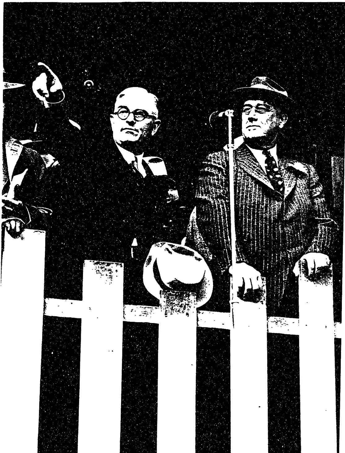
President Roosevelt views Grand Coulee Dam from Observation Point with Construction Engineer Banks.
