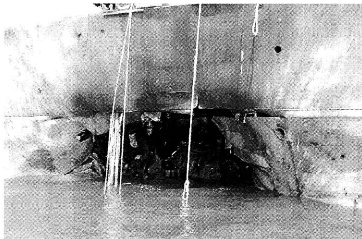
Figure A2: Close Up View of Above Waterline Damage
