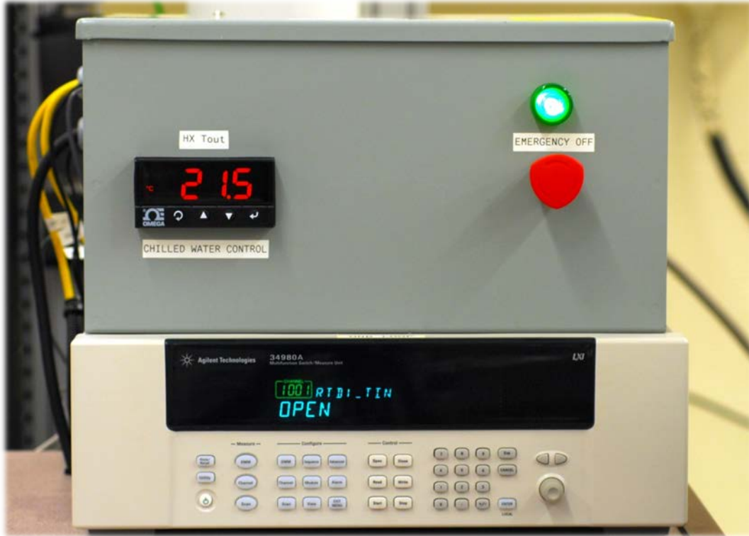
Figure 62: Data Acquisition System and Electrical Control Box.
