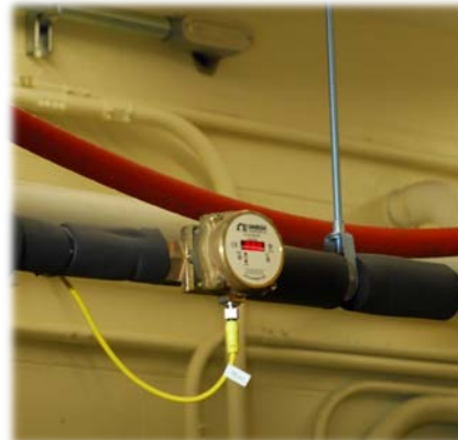
Figure 54: Vortex Flow Meter Installed in Primary Loop (left) and the Chilled Water Circuit (right).
