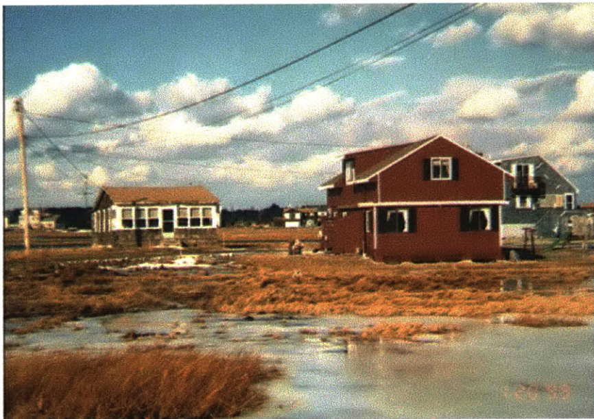
Figure 4.14 a and b Houses on the marsh in Hampton. Note the flow of water below the houses. These homes are all located below the syzygy tide line. (Photographs: J. Moore)
