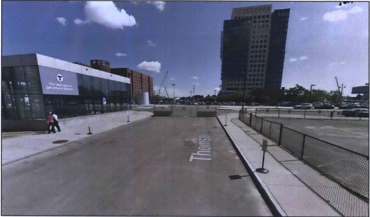
Figure 5-11: Dead-end at Thompson Place and Seaport Boulevard intersection
