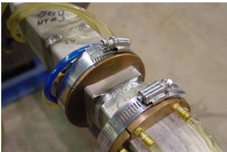
Fig. 3 Completion of auto-orbital welding
