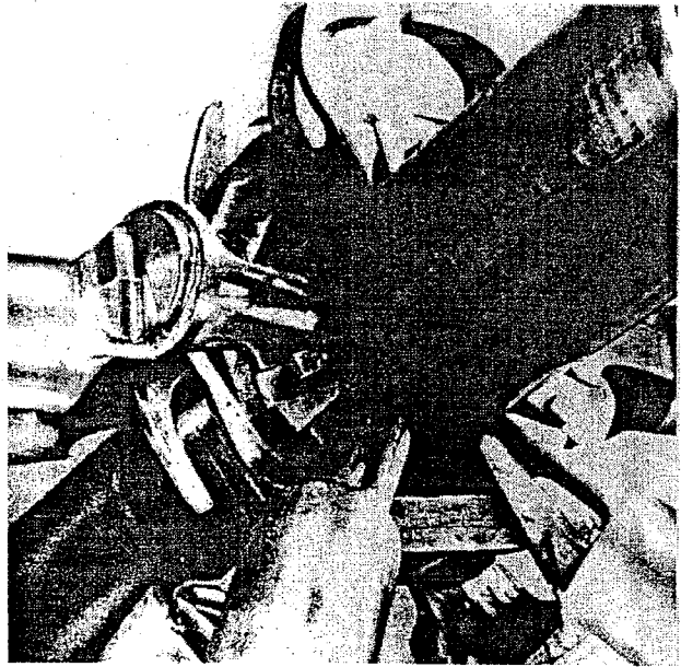
Fig 2.22e Tetrahedral system of space structure & joint for large hangar, K. Wachsmann Joint. Source: John Borrego, Space Grid Structures , pp.34-35.
