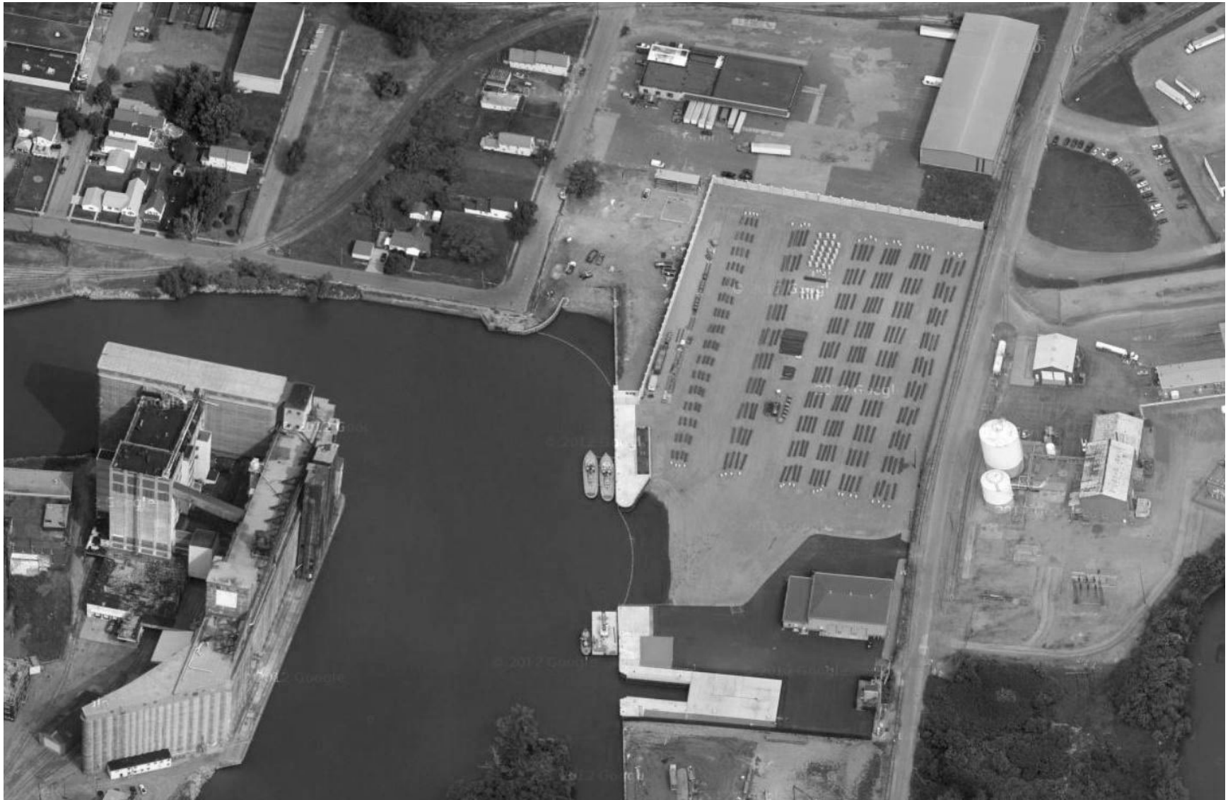
Recent site photo, with ice boom stored in rows on dry land, behind opaque fence along railroad Google Earth image
