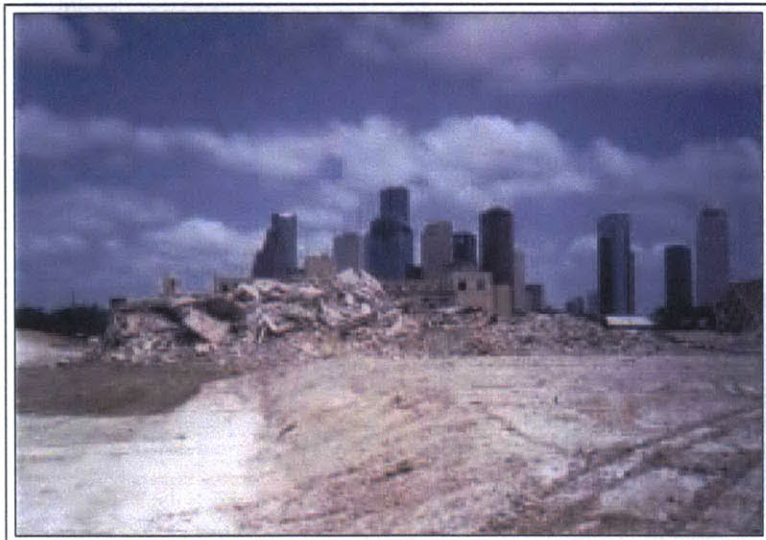
Demolition of city-owned hospital, May 1999
