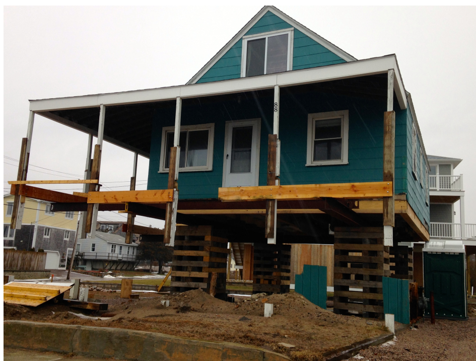
Figure 9: Home elevation construction on Atlantic Avenue in Westerly (2015)
