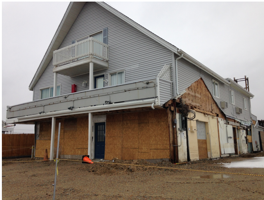
Figure 8: An elevated home along Atlantic Avenue in Westerly (2015)
