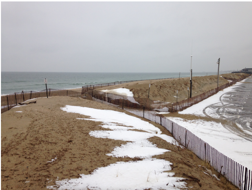
Figure 5: Rebuilt dunes along Atlantic Avenue in Westerly (2015)
