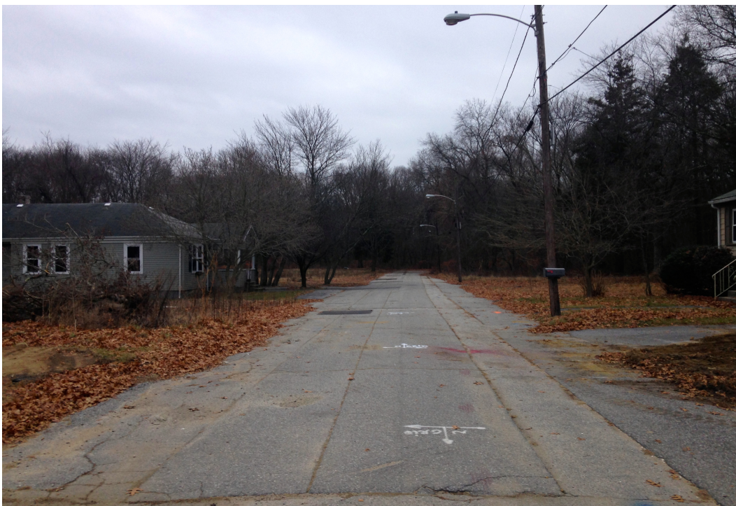
Figure 3: Perkins Avenue looking towards the Pawtuxet River (2014)
