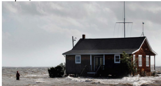
Figure 2: Images of Hurricane Sandy Aftermath, NOAA
