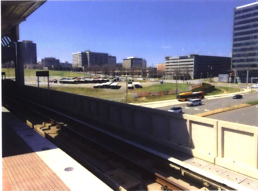
Figure 20: A concrete lot immediately northwest of Tysons Corner station
