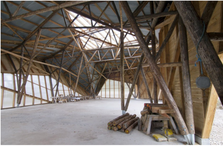
Fig. 3.1.1: “Big Shed,” interior view (Bennet, Self, and Randzio 2014)
