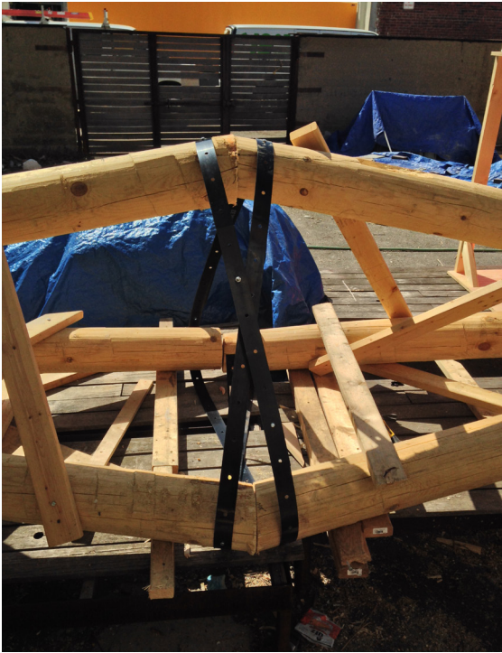
Fig. 4.2.12: Steel strapping at column mid-height.
