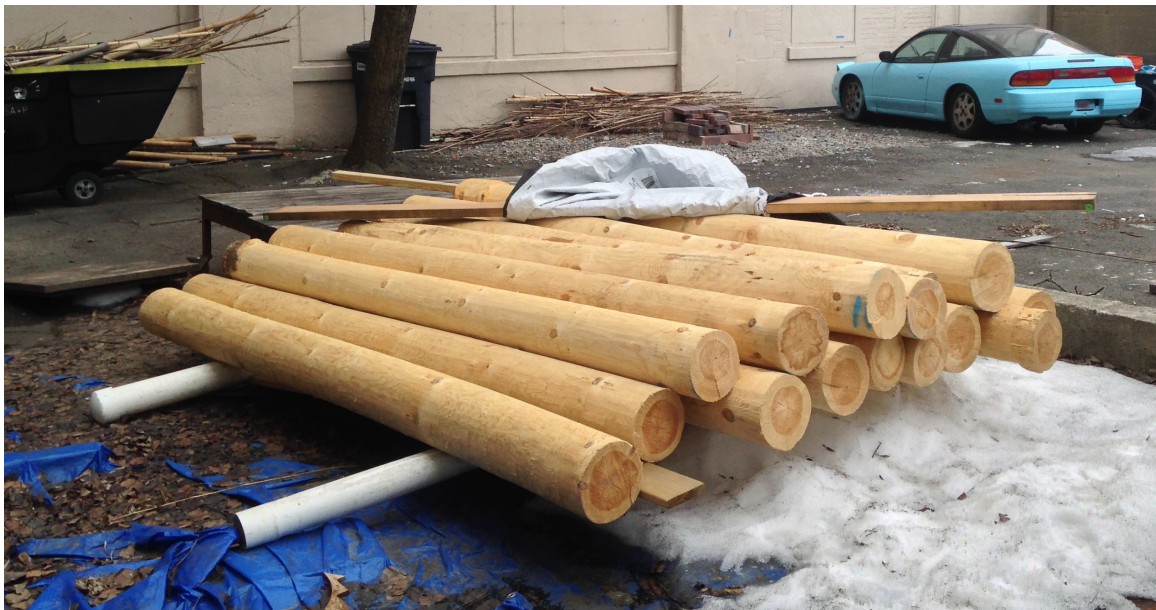
Fig. 4.2.8: 6" diameter 10' debarked, untreated red pine poles.
