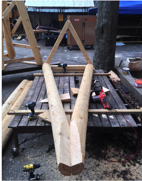
Fig. 4.2.10: Joining beveled ends of timbers.
