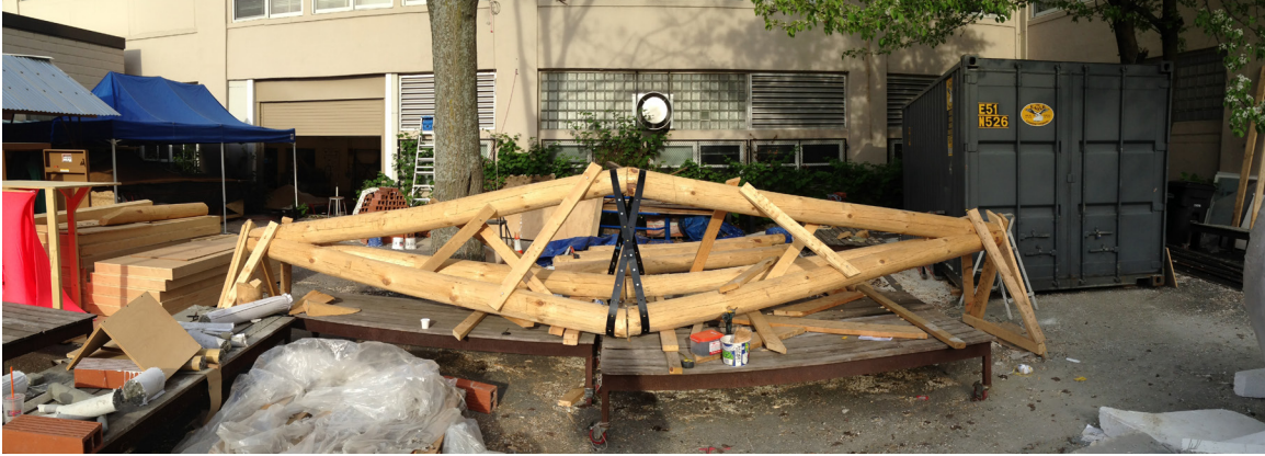
Fig. 4.2.16: Compound column in horizontal position being before post-tensioning.
