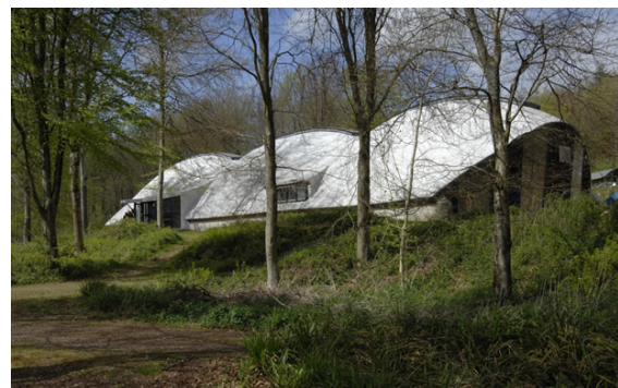
Fig. 3.1.4: Exterior of workshop at Hooke Park (Bennet, Self, and Randzio 2014)
