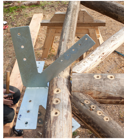
Fig. 3.1.2: Flitch plate connection (Evans 2011)
