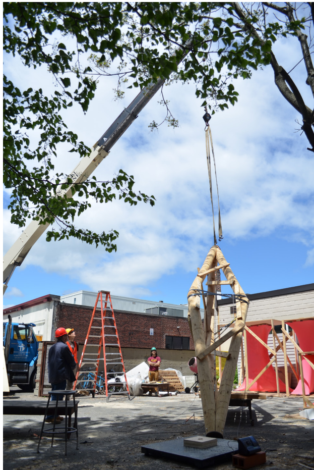
Fig. 4.2.17: Compound column being lifted by crane into standing position.
