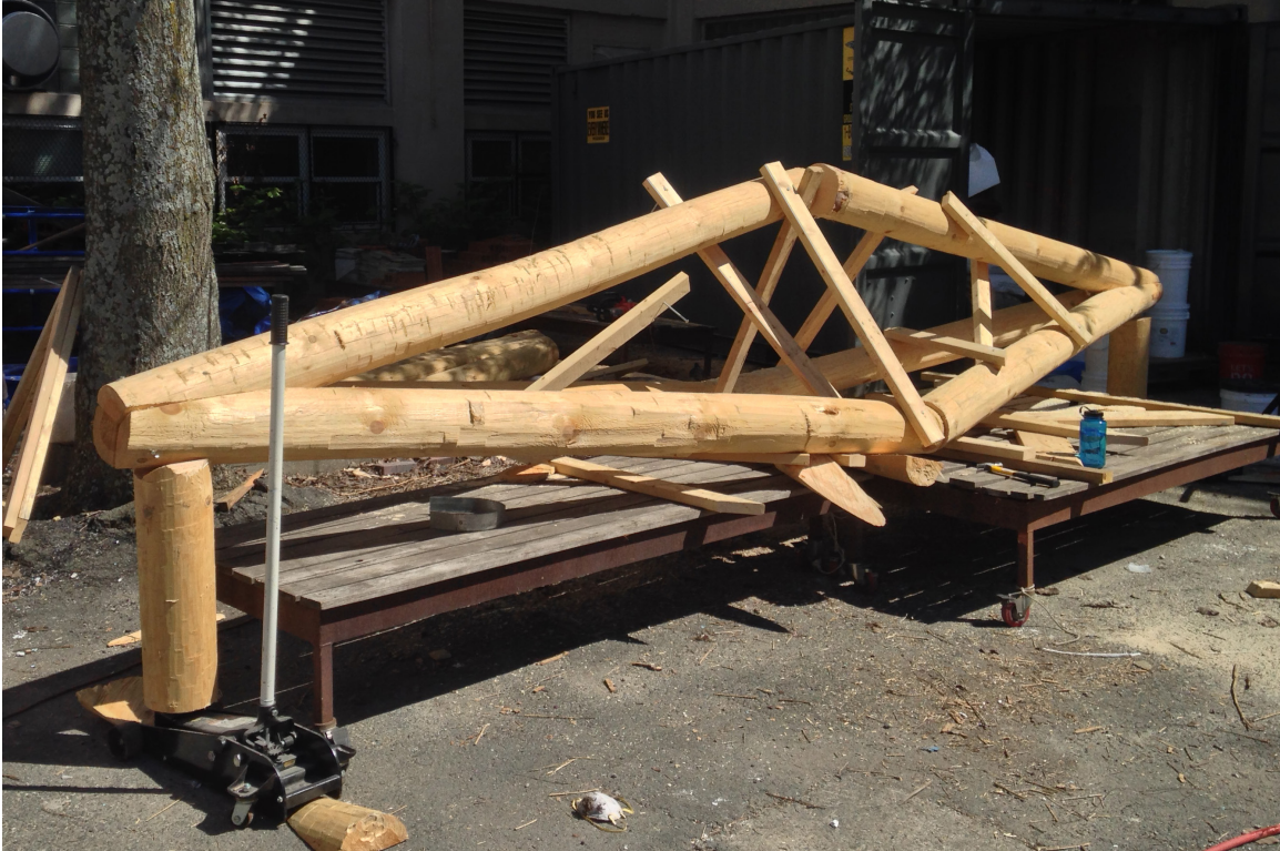
Fig. 4.2.11. Mating and aligning two halves of the compound column.
