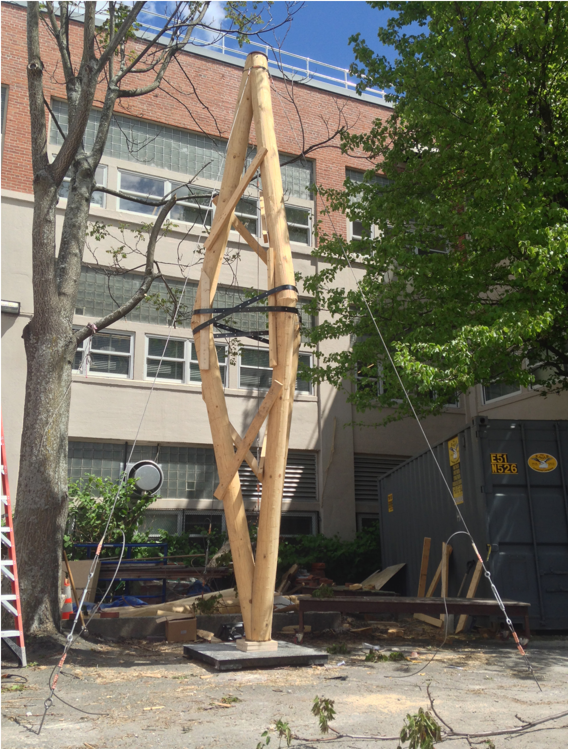
Fig. 4.2.18: Completed 20' compound column prototype (with temporary dimensioned lumber bracing).
