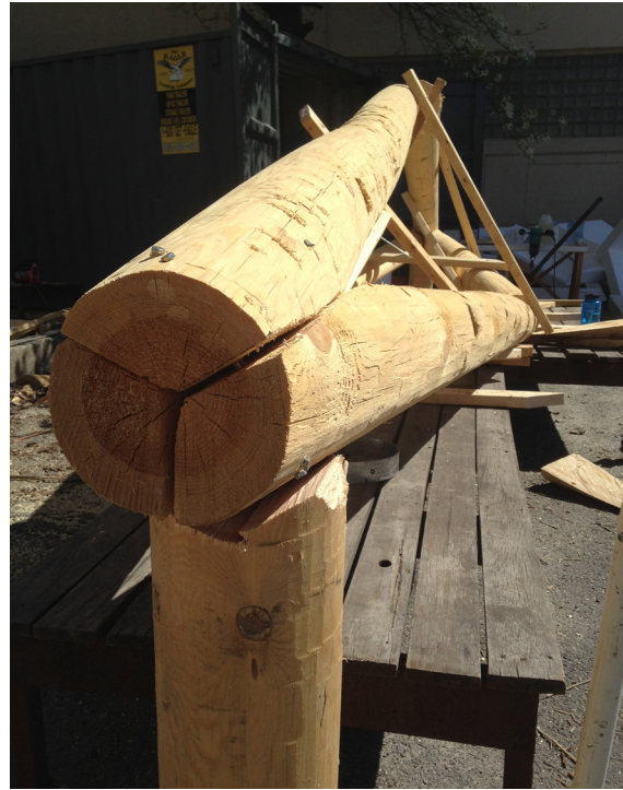
Fig. 4.2.13: End-node connection without steel cap.
