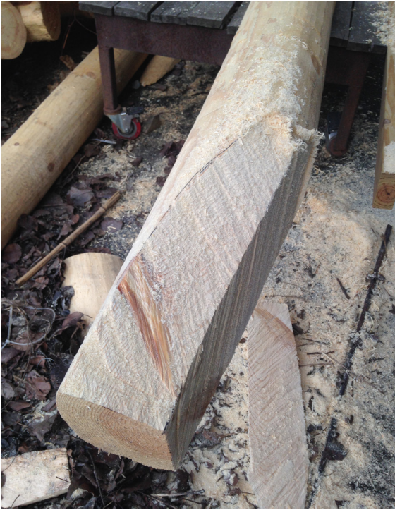
Fig. 4.2.9. Beveling of ends of timbers.
