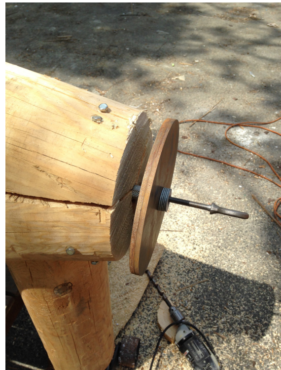
Fig. 4.2.15: Steel end-node connection assembly.
