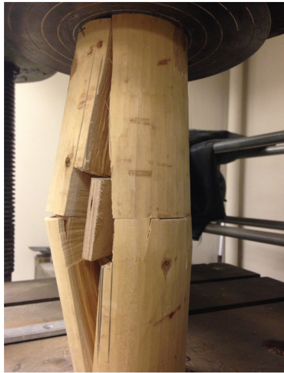
Fig. 4.2.4: Splitting failure in compression-only connection.
