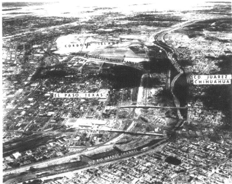
Figure 14. New Rio Grande Channel under construction, 1965.
