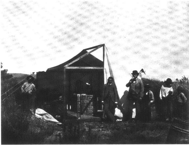
Figure 6. Surveying by zenith stars and moon culminations. An astronomical observatory constructed by the Mexican Boundary Commission. Near Tijuana, 1892.
