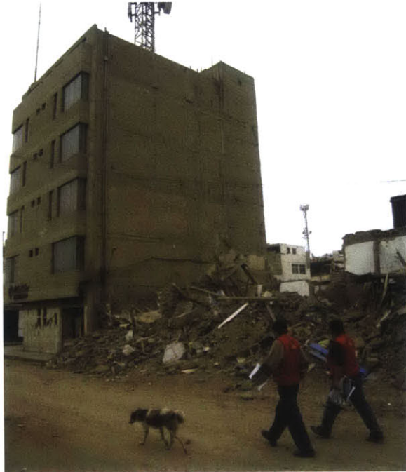
Fig. 2.1. Photograph taken in the aftermath of the 2007 Pisco, Peru earthquake (M8.0) by Blondet (2007). A six story confined masonry structure has survived with no damage whereas the building next to it completely collapsed.
