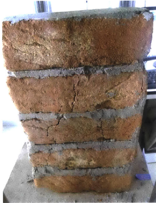
Fig. C.10. The crack initiated at the bottom of the second brick from the top and propagated in both directions.
