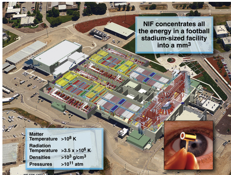
Figure 1.13. The NIF facility.
