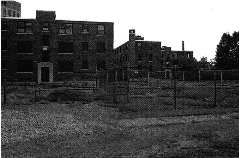
IMAGE 11. 73 DILAPIDATED NEWTOWNE COURT, CIRCA EARLY 1990'S
