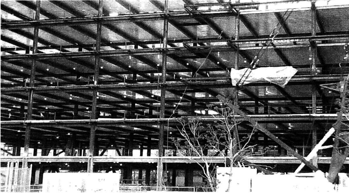
Illustration 6. Amgen's new 285,000 square foot research facility under construction
