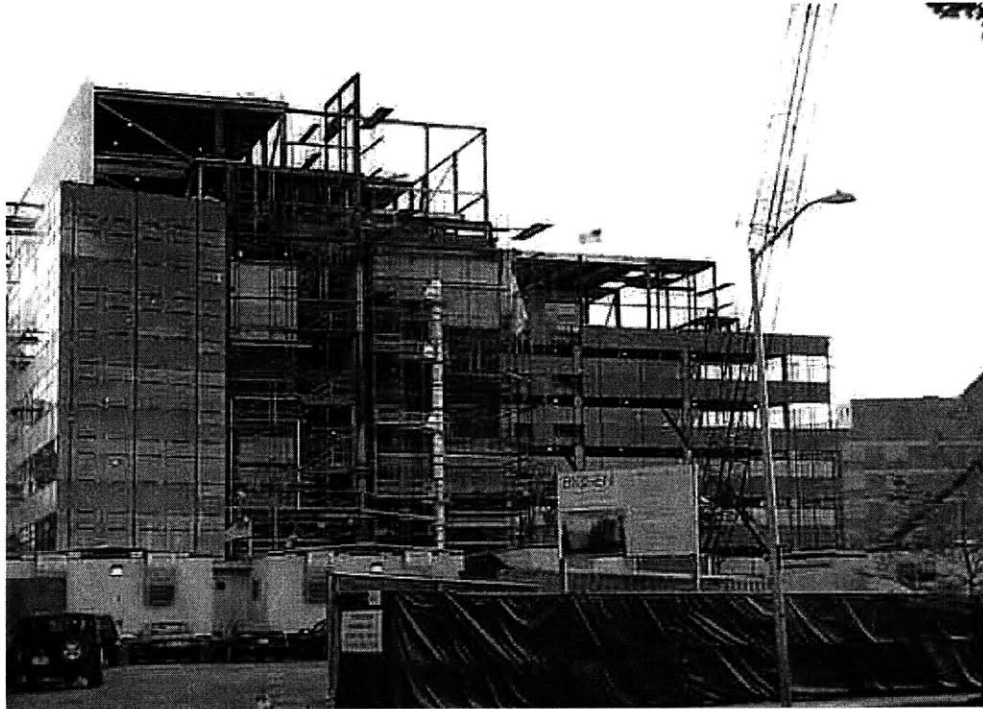
Illustration 3. Biogen's new research facility under construction
