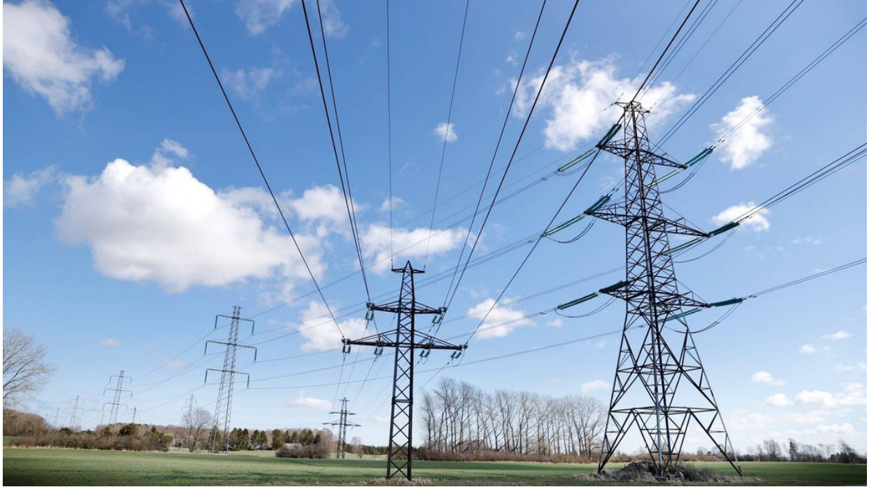
Figure 42: Transmission towers to be demolished in Roskilde, Denmark. (© Jens Dresling)
