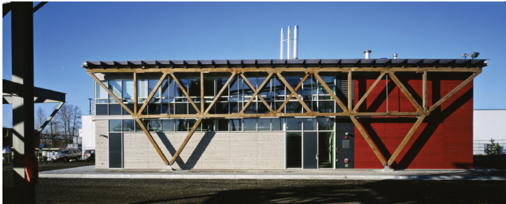
Figure 2: The City of Vancouver Materials Testing Laboratory uses materials from local demolitions. By Martin Tessler, courtesy: Perkins+Will.
