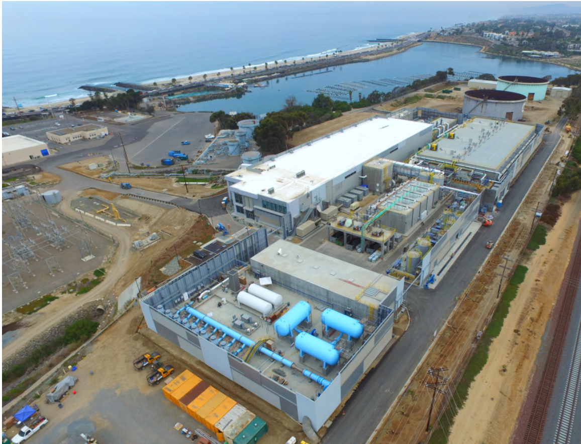
Figure 5.2: The Carlsbad desalination plant
