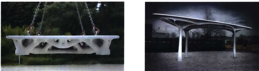
Figure 9: Built concrete structures designed with topology optimization
