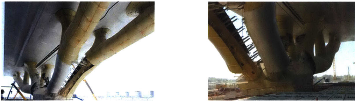
Figure 4: Qatar National Convention Center under construction; photos borrowed from Matsuuro Sasaki
