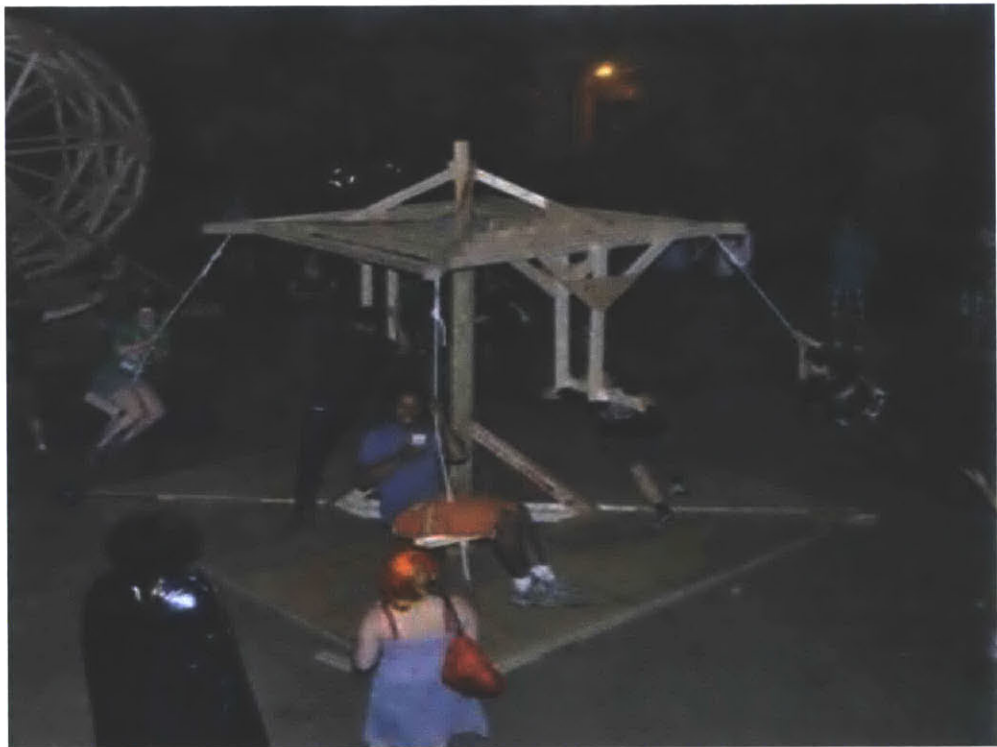
Figure 22: Completed ride in operation. Slightly left and right of center, two pushers are pictured. Despite the clear difference in weight and size of the riders on left and right of the picture, all swings are at the same angle from vertical. A small deflection in the upper cantilevered beam is visible for the left rider; it is less than the maximum predicted 8". Riders sit according to Section 2.2.5.
