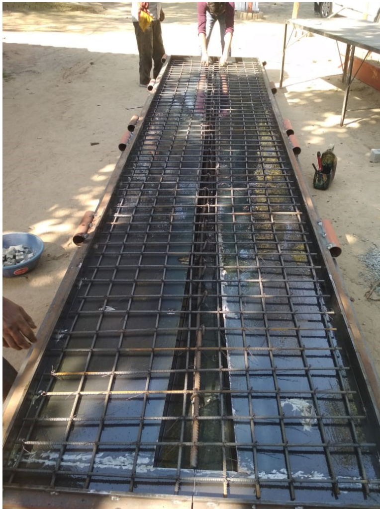
Figure 79 Rebar placement within prototype mold
