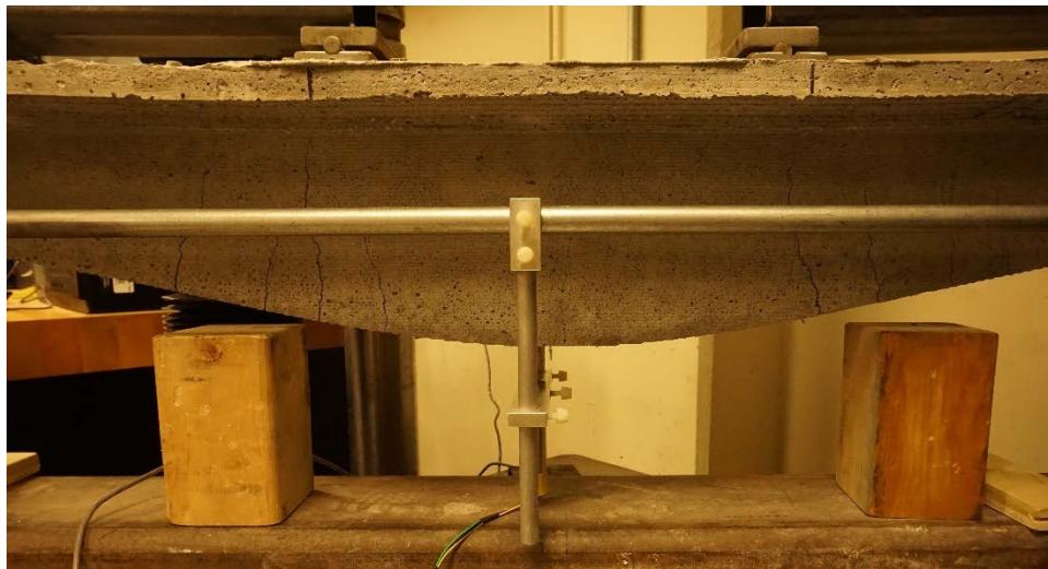
Figure 72 Close up of Slab 2 after loading shows flexural cracks near midspan
