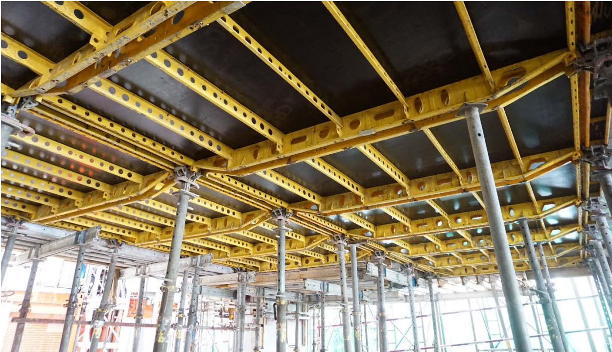
Figure 103 Assembled formwork for flat concrete slab supported by steel poles
