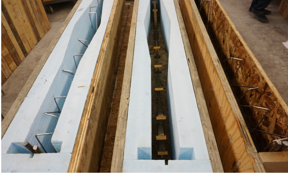
Figure 37 Shaped beam formwork and reinforcement
