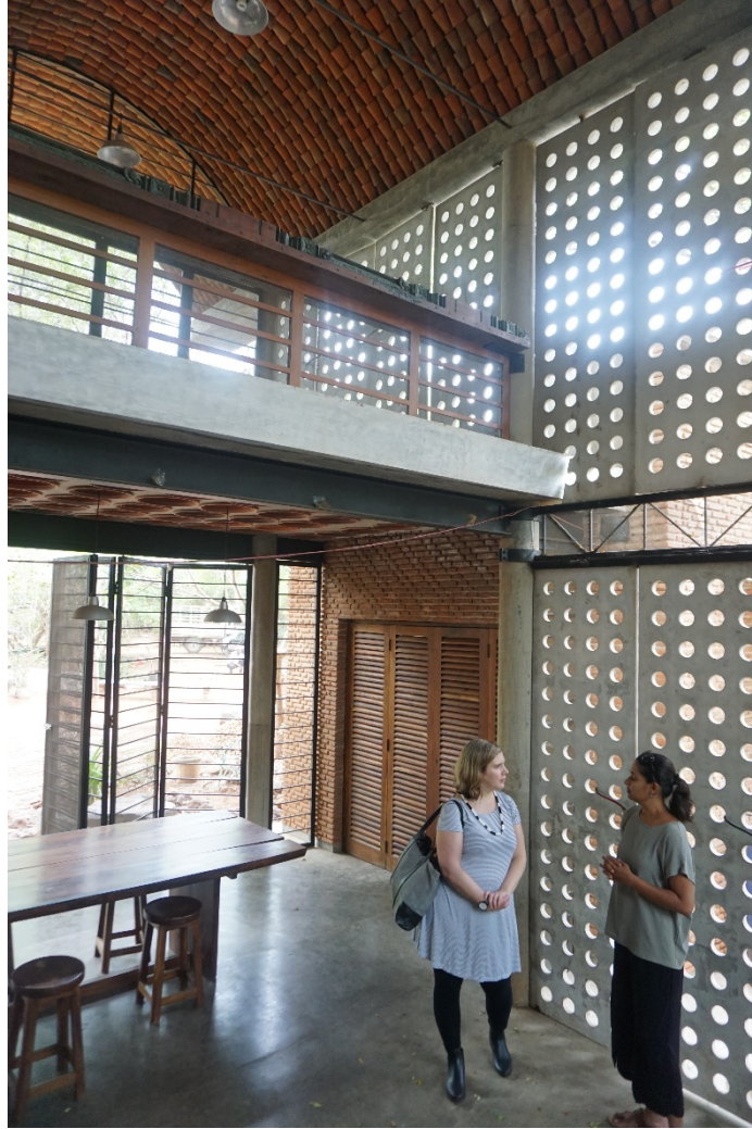
Figure 14 Ferrocement panels, vaulted roof, and filler slab in Wall house, Anupama Kundoo, Auroville, 2000
