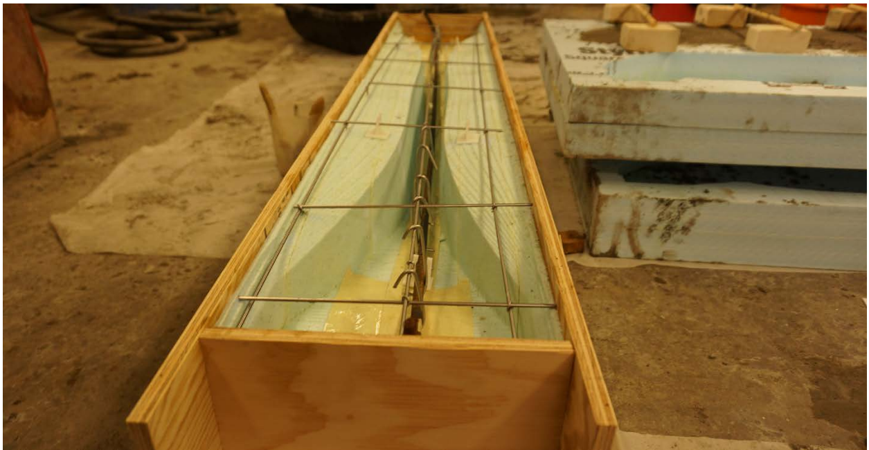
Figure 97 CNC milled foam, plywood box, and steel reinforcement of shaped slab prototype
