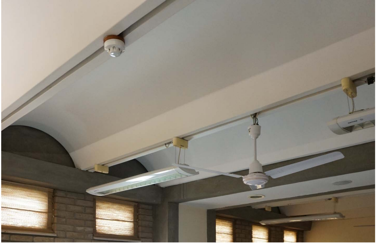
Figure 116 Semi-circular ferro-cement channels, New Delhi, courtesy of Development Alternatives (DA)
