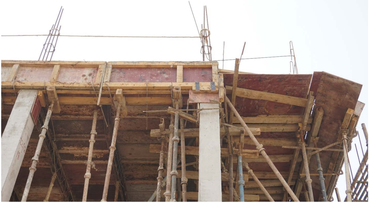
Figure 110 Formwork for cast-in-situ flat slabs
