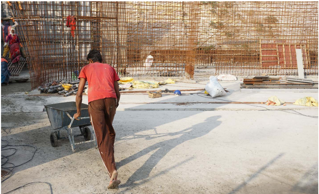
Figure 107 Construction worker carting ready-mix concrete to pouring location
