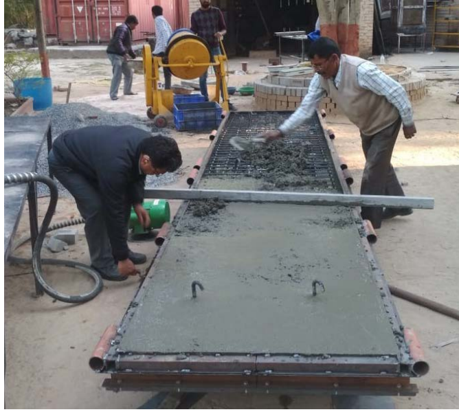
Figure 80 Concrete casting and finishing
