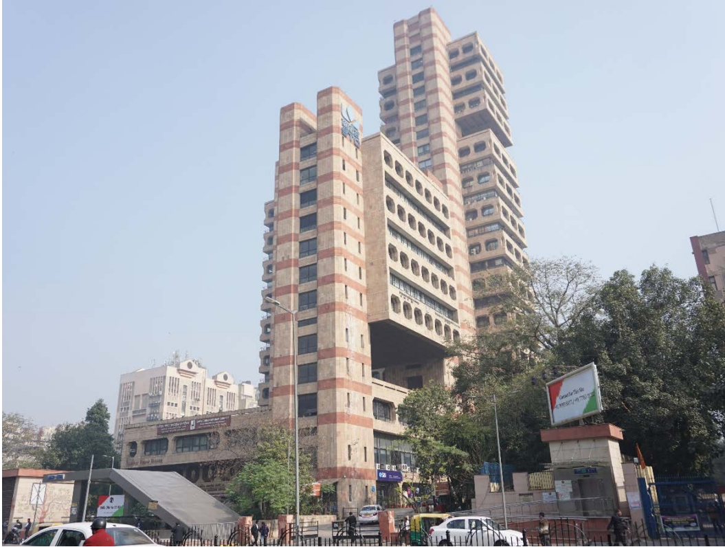
Figure 124 Suspended floors at State Trading Corporation by Raj Rewal and Mahendra Raj, New Delhi, 1988
