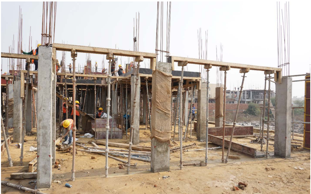
Figure 109 Cast-in-situ concrete columns and formwork for beams
