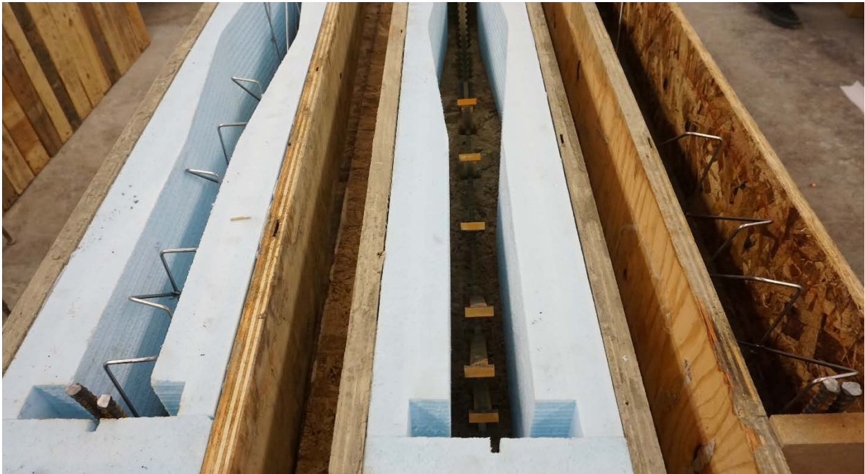
Figure 93 CNC milled foam and plywood boxes for shaped beams
