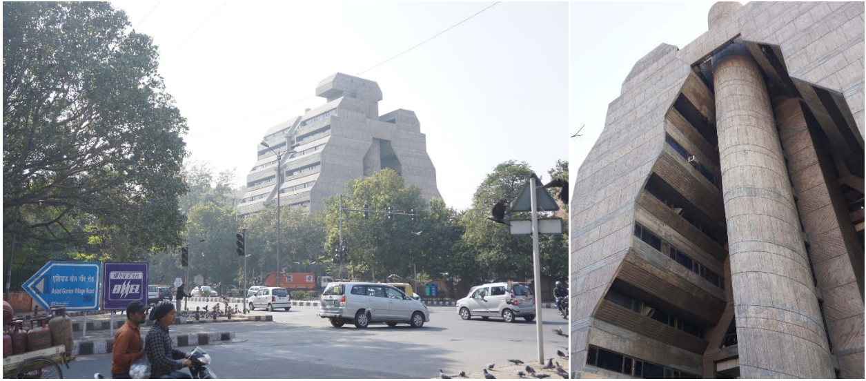
Figure 126 Post tensioned leaning towers of NCDC by Kuldip Singh and Mahendra Raj, New Delhi, 1980
