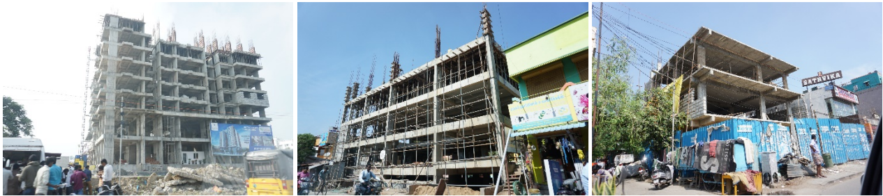
Figure 1 Informal survey of common construction practices in Indian cities
