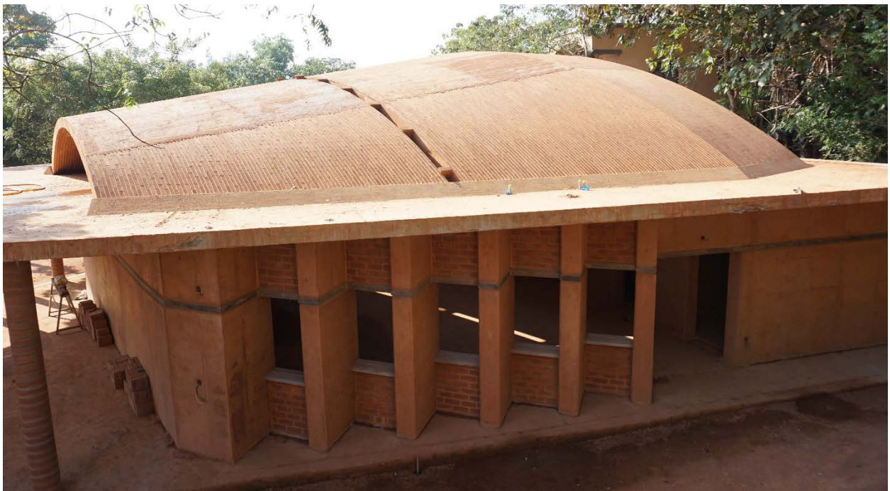
Figure 115 Exterior of 15m-span conical vault, Pondicherry, courtesy of AVEI
