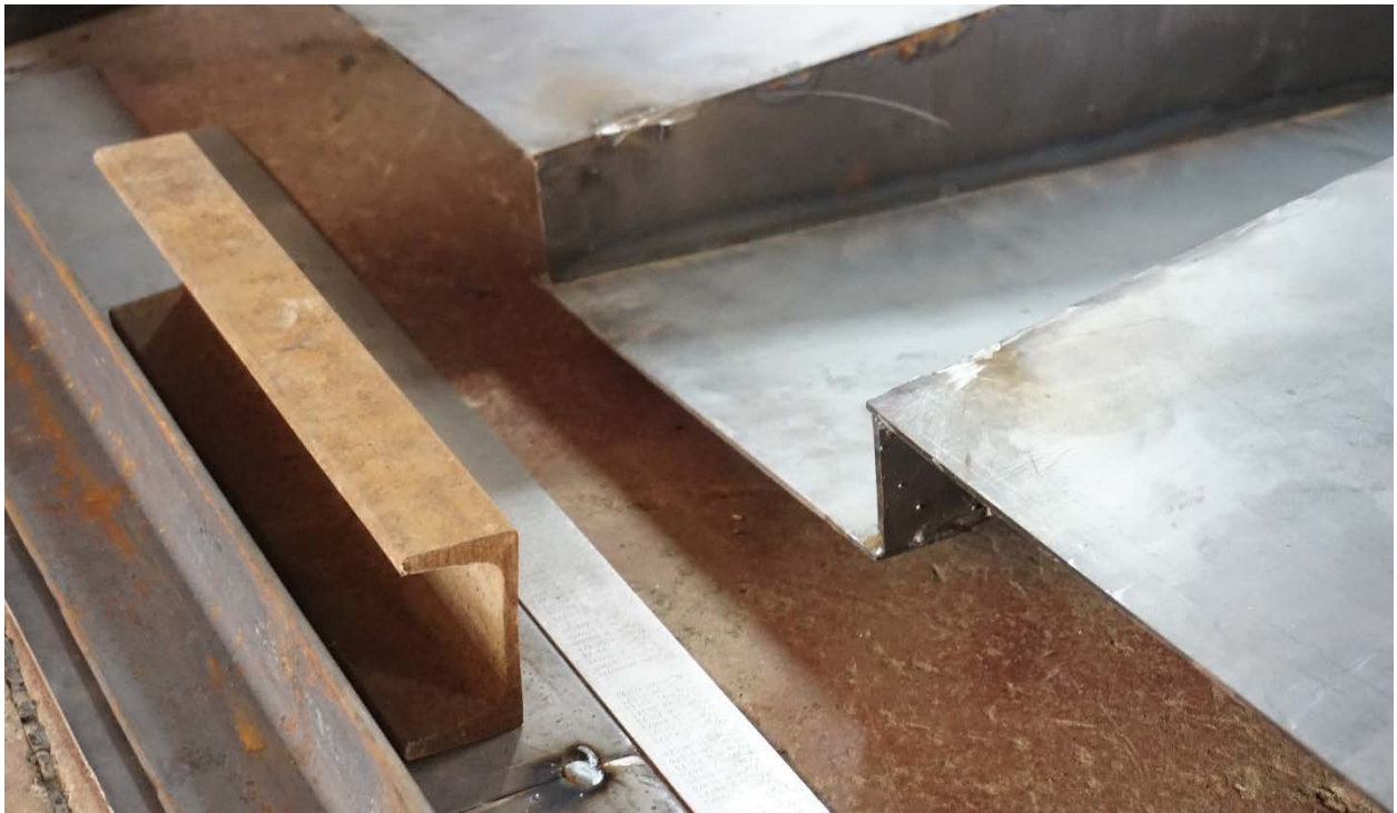
Figure 77 Close up of sheet metal formwork showing manually welded joints
