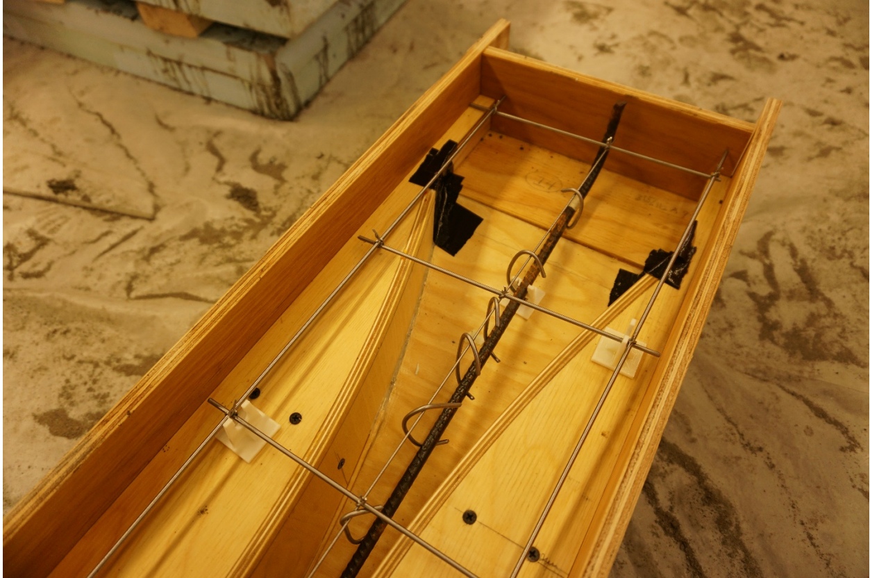
Figure 98 Bent wood and steel reinforcement for shaped slab prototype
