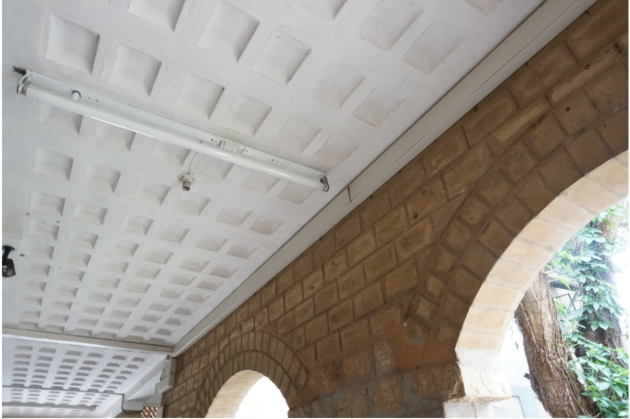
Figure 120 Standard filler slab, courtesy of Indian Institute of Science (IISc)
