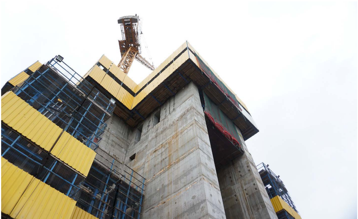
Figure 105 Auto-climbing system used in construction of vertical core
