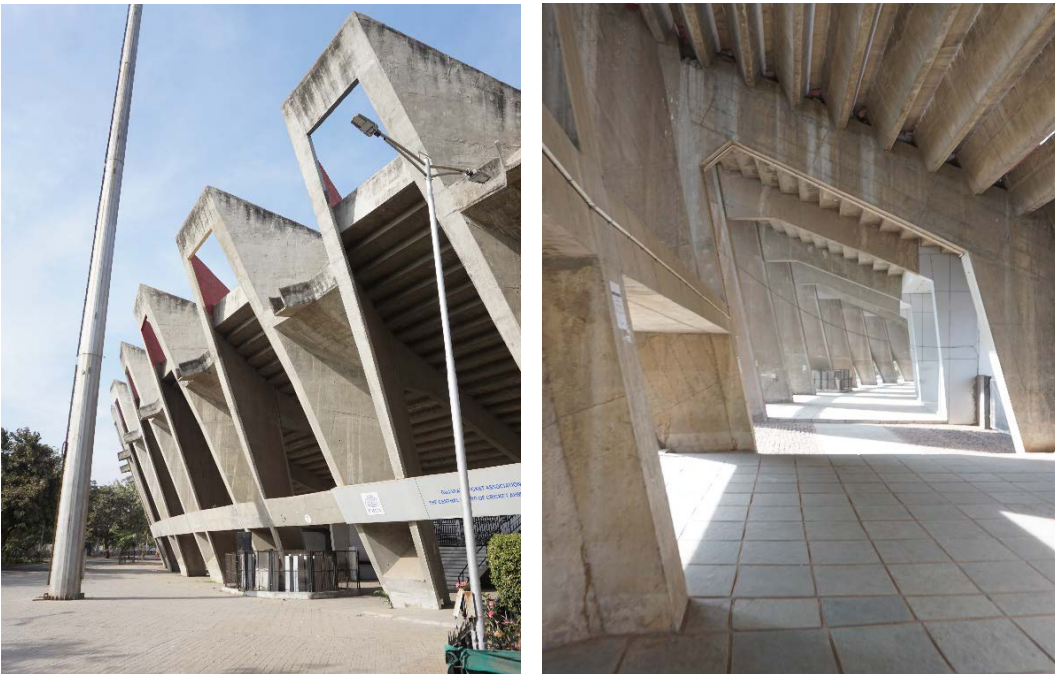
Figure 125 Folded plates and beams at Municipal Stadium by Charles Correa and Mahendra Raj, Ahmedabad, 1960
