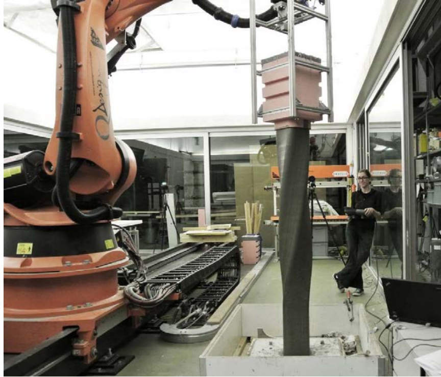
Figure 26 Concrete pillar built using Smart Dynamic Casting/slip-forming, ETH Zurich
