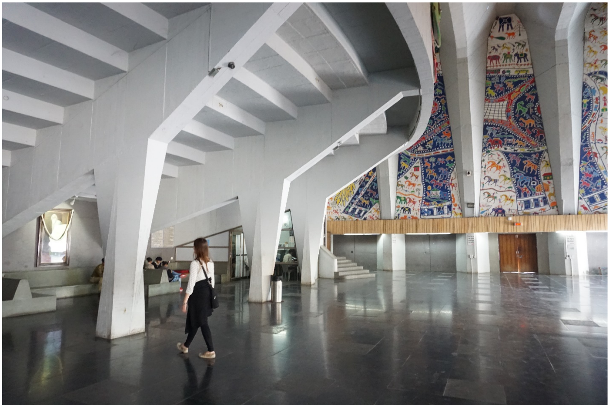
Figure 127 Folded plates and twisted columns of Tagore Hall by BV Doshi and Mahendra Raj, New Delhi, 1965
