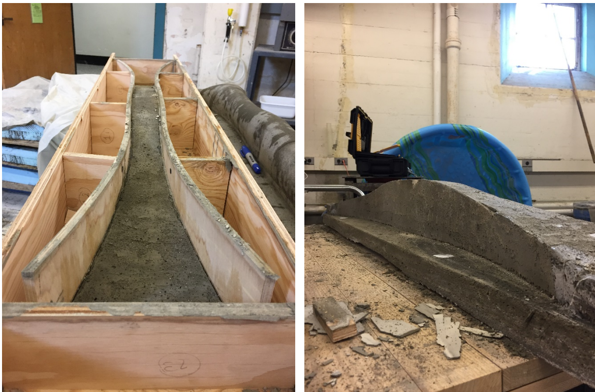
Figure 101 Close up of bent wood formed shaped slabs
