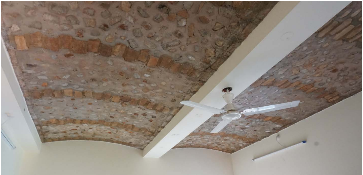
Figure 121 Jack arch using construction waste and low-carbon concrete, courtesy of IISc
