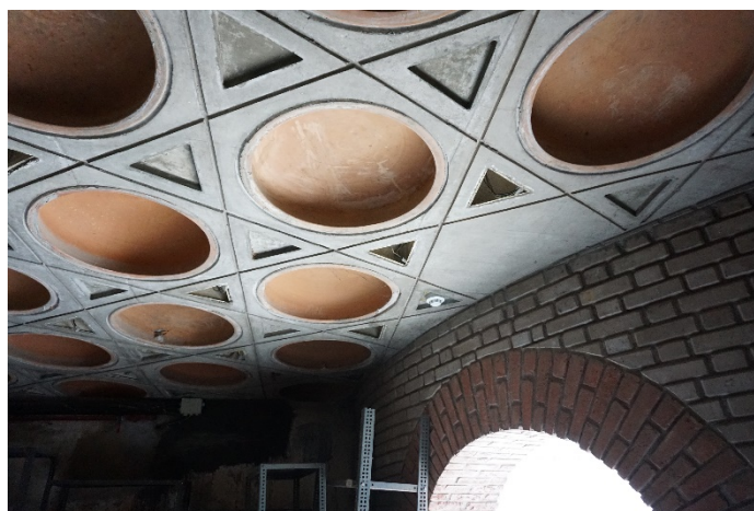
Figure 13 Filler slab; Development Alternatives Headquarters, Ashok B. Lall Architects, New Delhi, 2014
