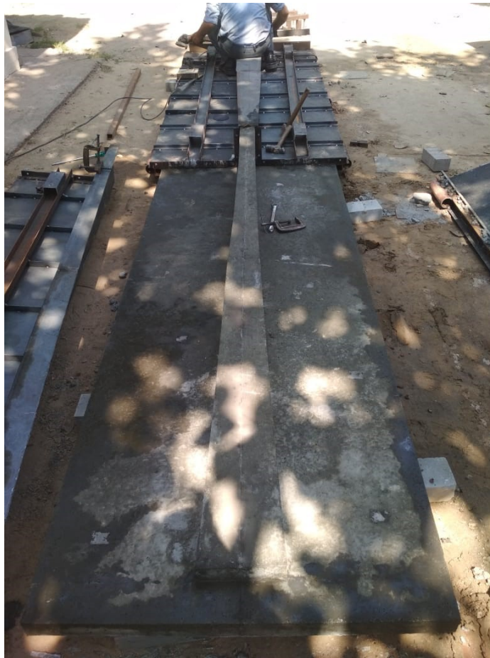
Figure 81 Demolded slab with parts of reusable formwork lying beside it
