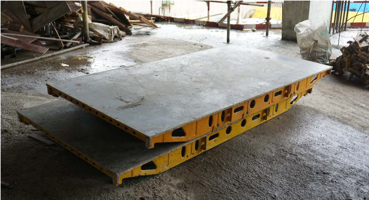
Figure 102 Imported formwork for flat-slab construction, courtesy of Larsen & Toubro
