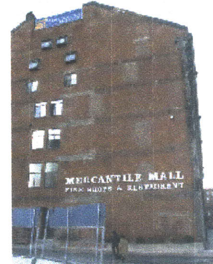
(6) Buildings constructed before the highway were often modified to deflect noise and pollution. Now they must reconvert to face a new amenity.
