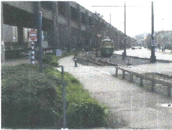
(4) The viaduct stands as a physical and perceptual wall between the waterfront and city center.
