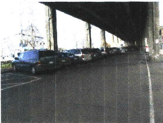
(3) Space under the Viaduct is almost entirely used for a single row of angled surface parking.
