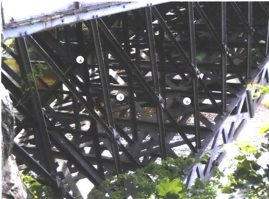
Figure 3.6: Lateral components of Craigellachie Bridge, perspective view closeup (Lane 2017)
