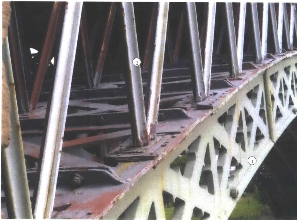
Figure 3.13: Mythe Bridge – lattice-rib connections, covering plates, external rib (Lane 2017)
