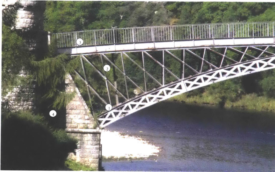
Figure 3.4: Vertical components of Craigellachie Bridge, closeup view (Lane 2017)
