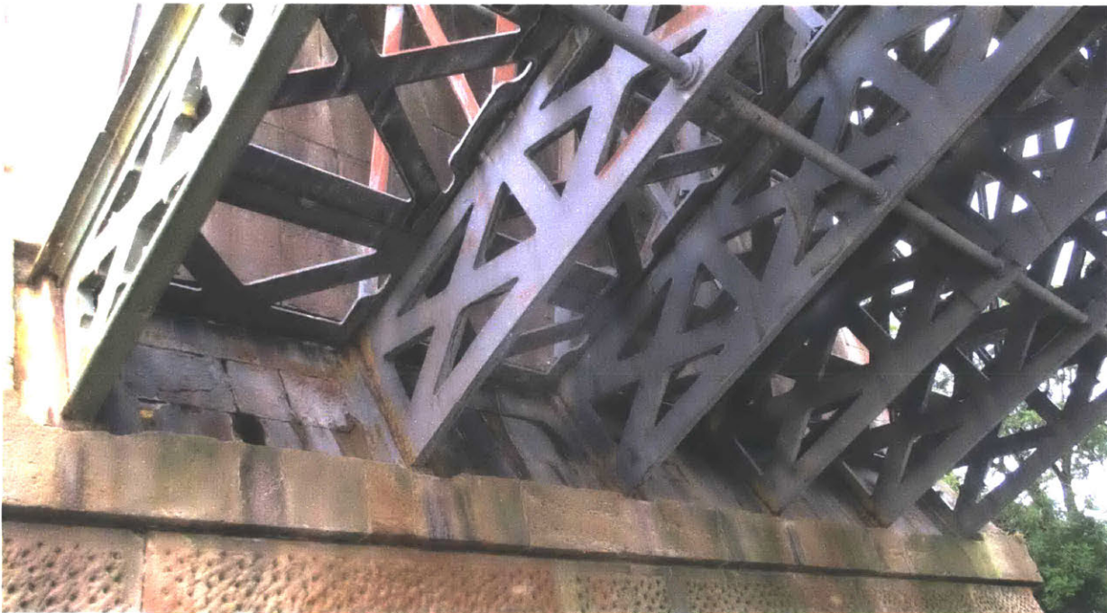
Figure 5.11: Springing plate – Mythe Bridge (Lane 2017)
