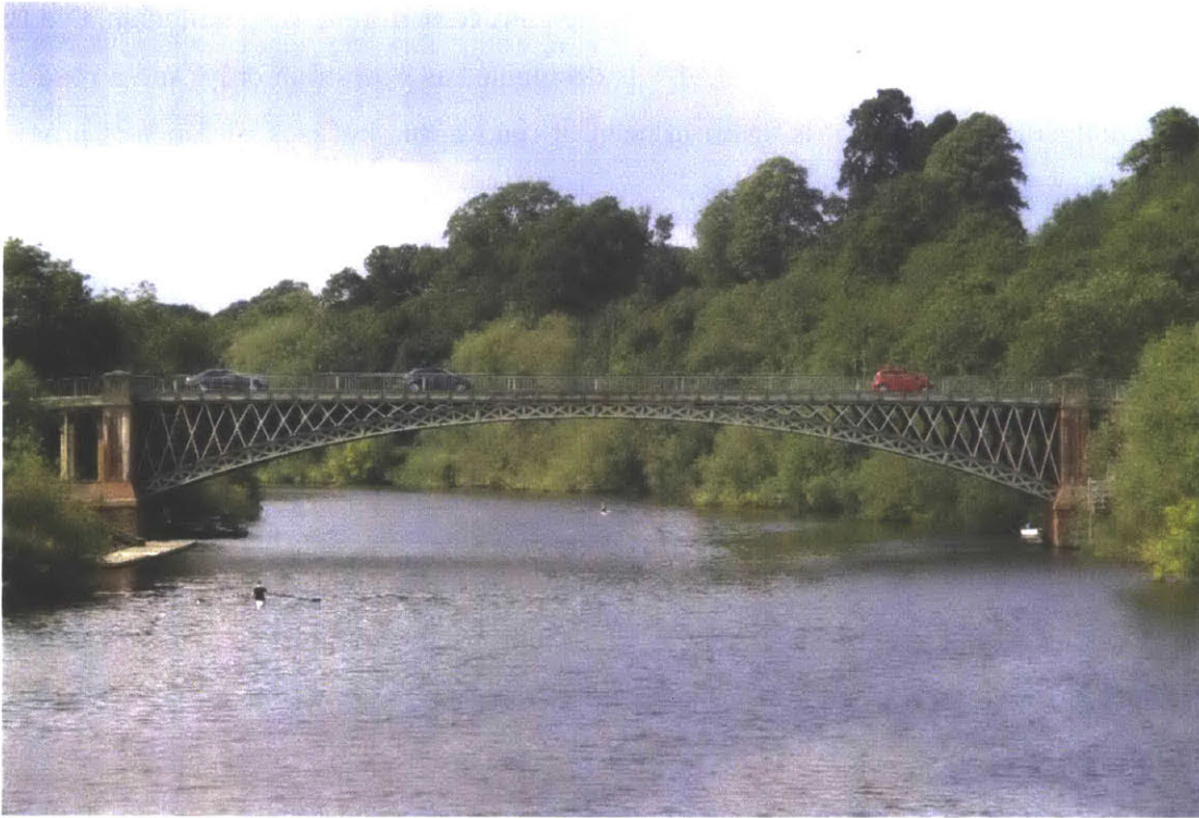
Figure 3.9: Mythe Bridge, full elevation (Lane 2017)
