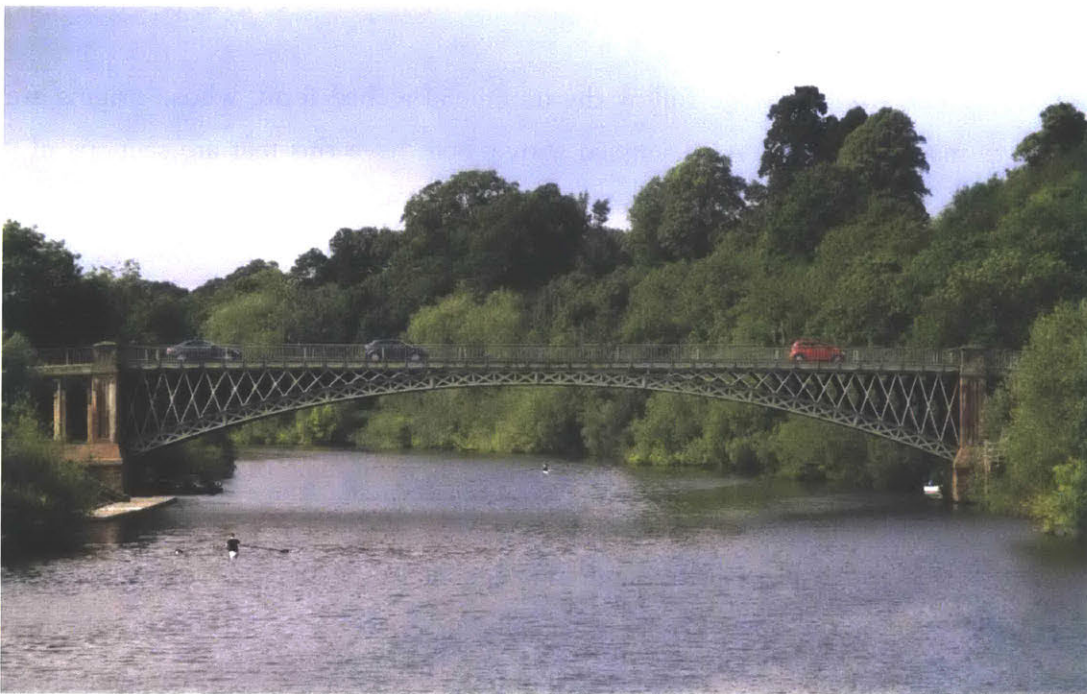
Figure 5.2: Mythe Bridge (Lane 2017)
