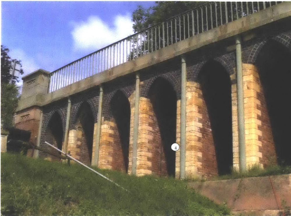
Figure 3.14: Mythe Bridge – abutment (Lane 2017)
