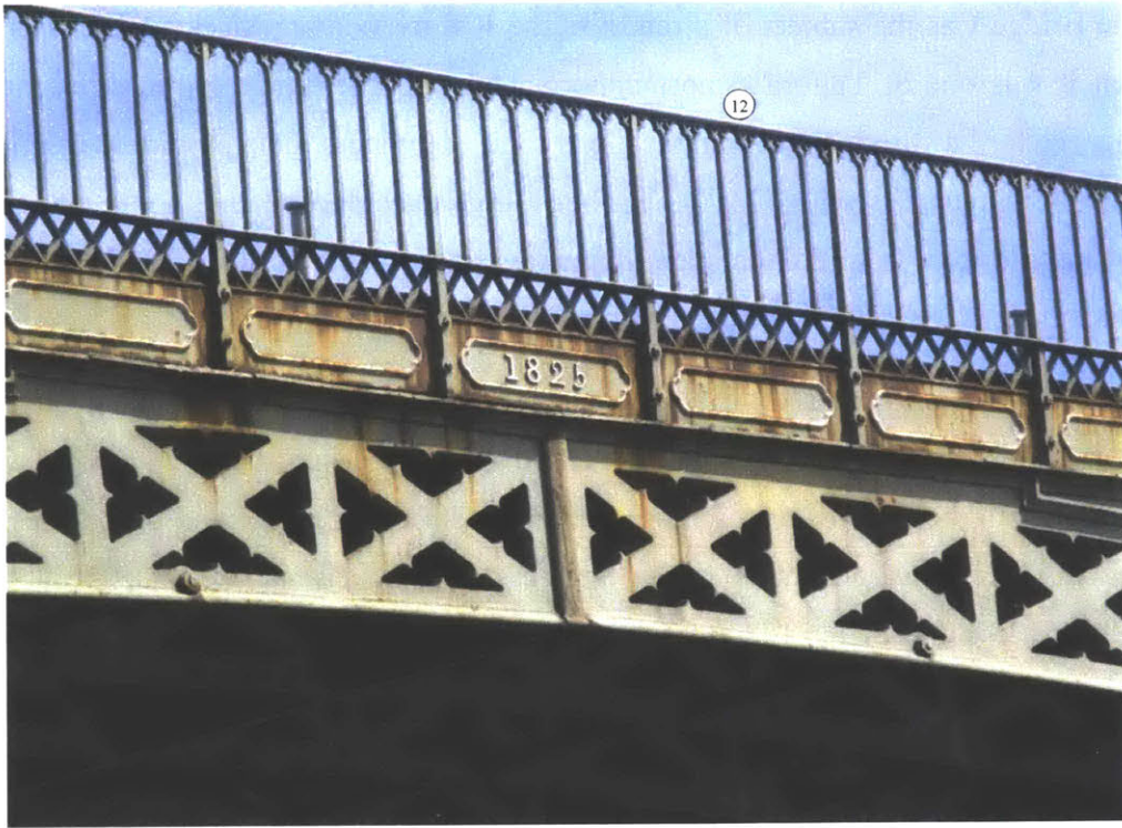
Figure 3.16: Mythe Bridge – original railings, skirting plates, and ribs (Lane 2017)
