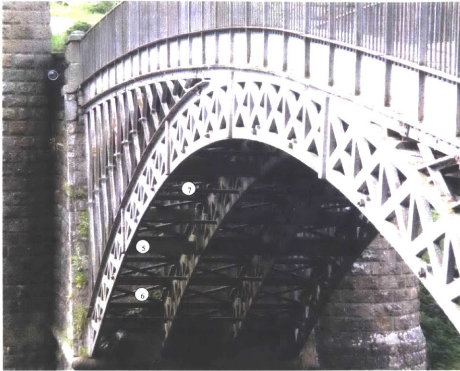
Figure 3.5: Lateral components of Craigellachie Bridge, perspective view (Lane 2017)
