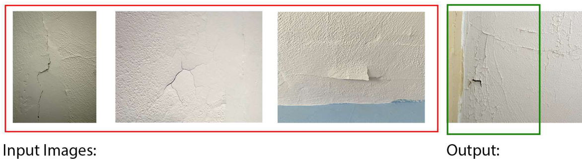
Figure 3. Output from the TensorFlow-based damage detection model, highlighting areas of cracks in a previously unseen image. The red highlight outlines some of the training images that were provided as input. The green bounding boxes are drawn around detected crack regions on a test image.
