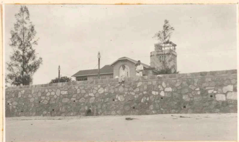
Embankment in front of the Palace
