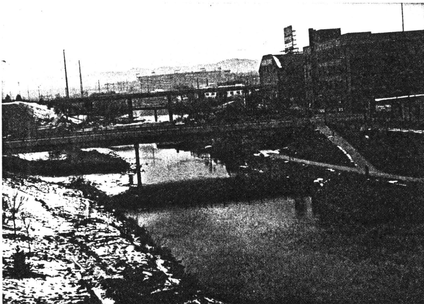
View of Platte River from the 16th Street viaduct.
