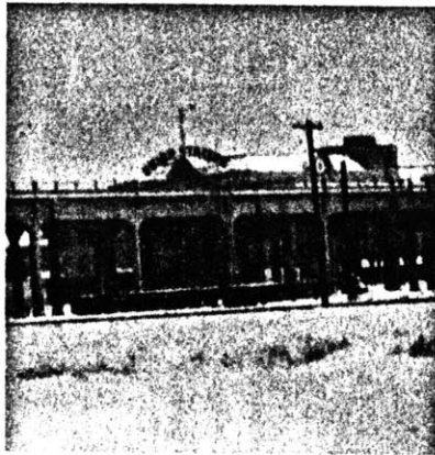
The existing 16th Street viaduct. The viaduct was constructed nearly 60 years ago to cross the railyards and connect neighborhoods at a higher elevation northwest of Denver with the central business district of Denver. The viaduct, which is structurally unsound to continue its present use, acts as a pedestrian as well as vehicular link.
