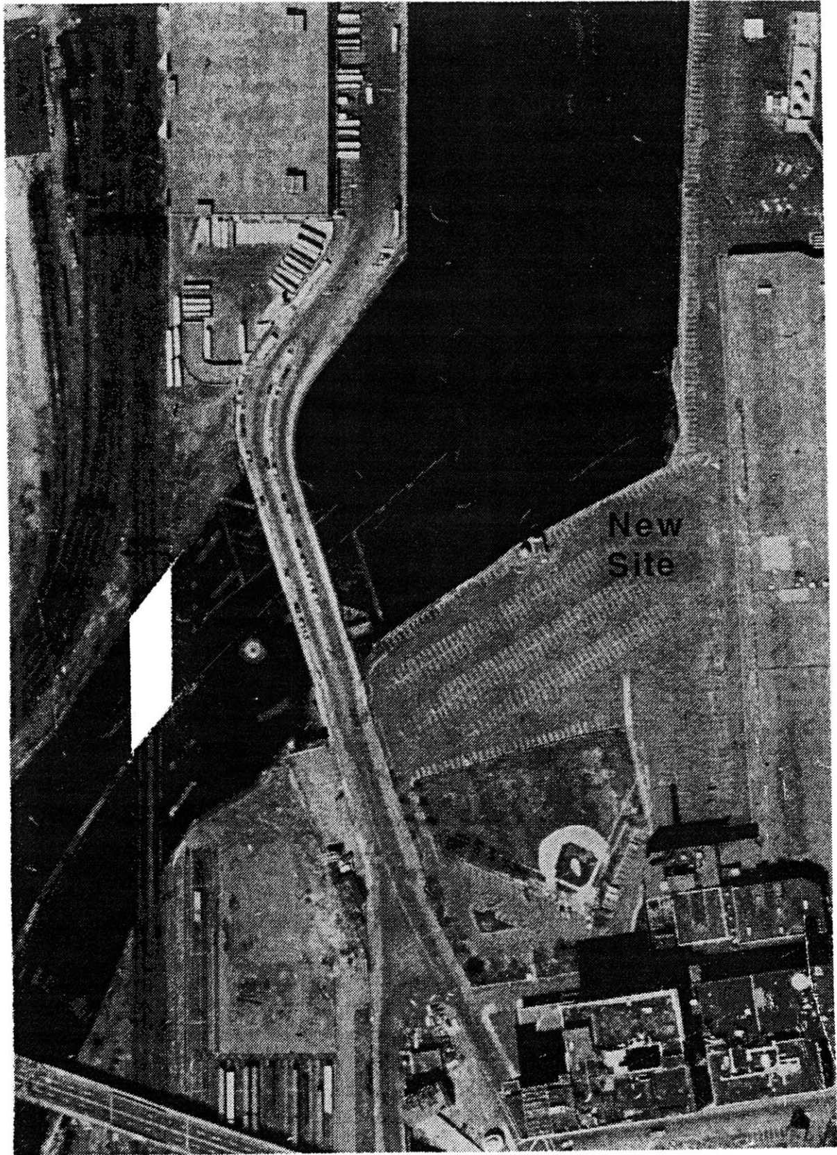
fig. 23 Building site in relation to the bridge
