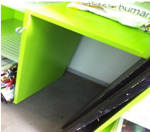
Figure 5-10. Sensor No.21 on 2F (behind the desk)
