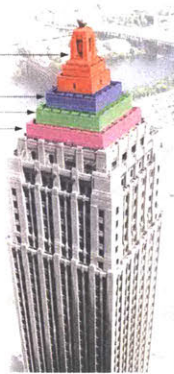
The KDKA-TV Weather Beacon. The Gulf Tower, Pittsburgh, PA. Weather information with floor by floor breakdown. 39th floor: wind speed; 40th floor: humidity; 41st floor: precipitation; 42nd - 44th floor: temperature. (DiCello, 2016)
