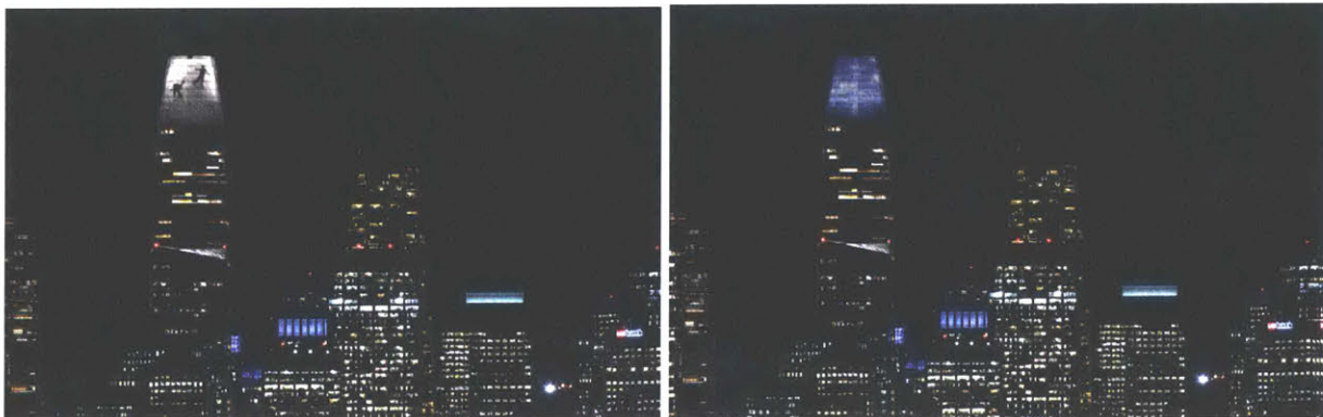
Salesforce Tower, San Francisco. 11,000 LEDs were installed on the top six floors, displaying the daily life story recorded by multiple cameras placed around San Francisco. (Campbell, 2017)
