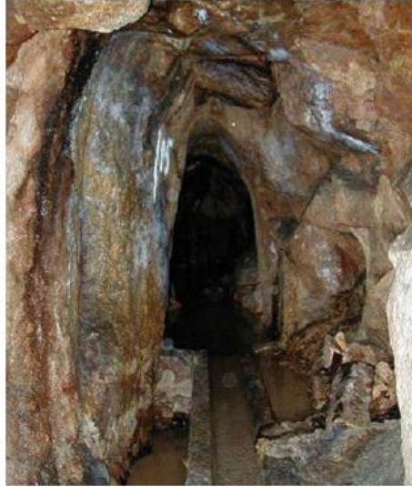
Figure 33 Man-made tunnels (“minas”) in Porto, Portugal (from Forrest, 2006)
