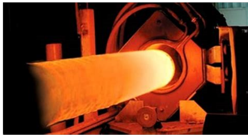
Example of induction reheat furnace
