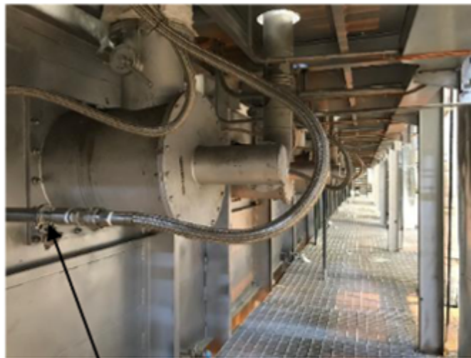
O 2 lance retrofit next to existing burners
