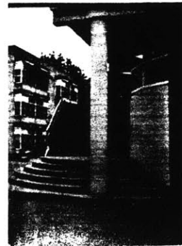
Herman Hertzbergers Appollo School in Amsterdam. The column is in the middle of the stairs.
