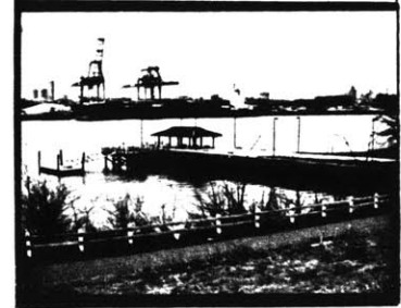
view of Massport Piers from between buildings in Jeffries Point . The pier was raised at its connection point with the land to allow for turning trains.
