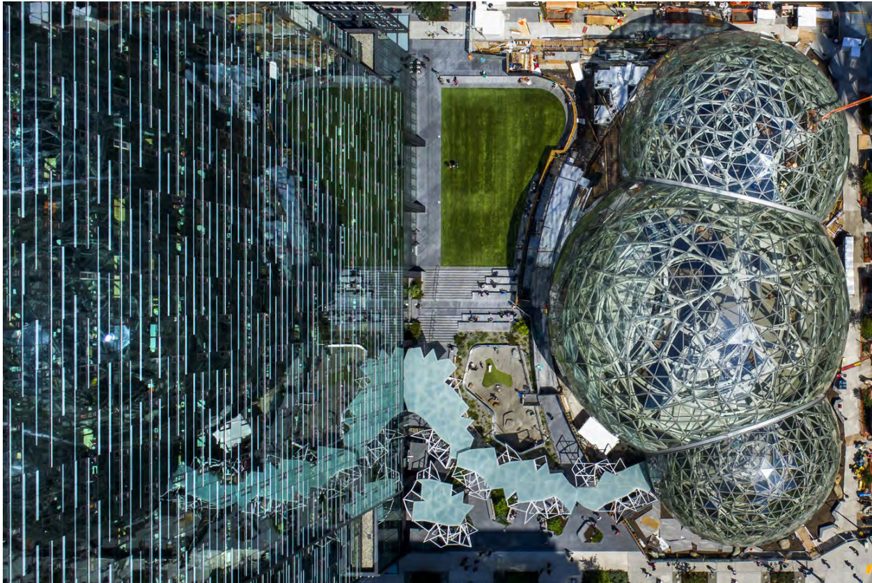
FIGURE 1.1 Designed by NBBJ, the bespoke “Amazon Spheres” building was completed in 2018.
