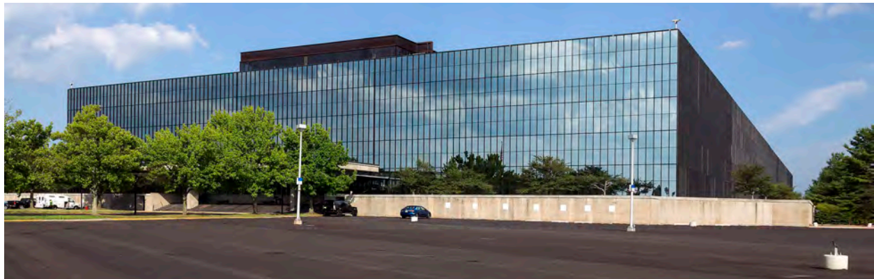
FIGURE 2.13 In pure Modernist expression, the exterior of Bell Labs Holmdel Complex resembles a large mirror box.
