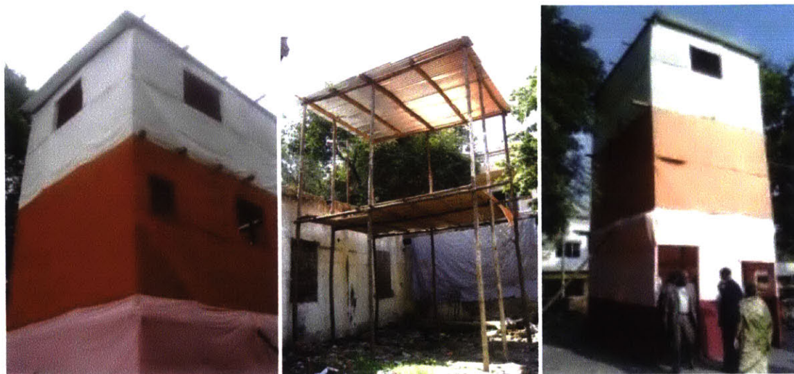
1:1 model house mockup erected onsite -photographs- courtesy Prasanna Desai
