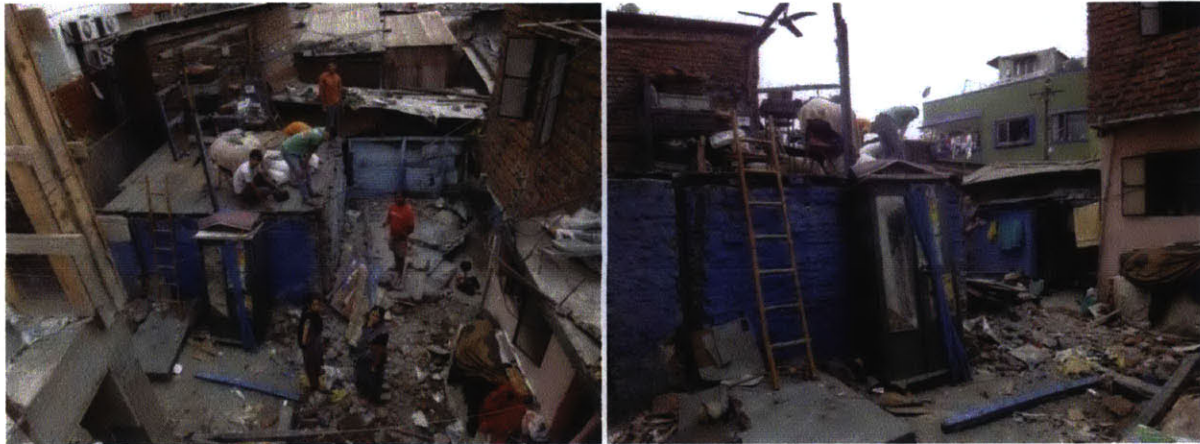
Self-demolition work in progress, Mother Teresa Nagar -photographs- courtesy Prasanna Desai
